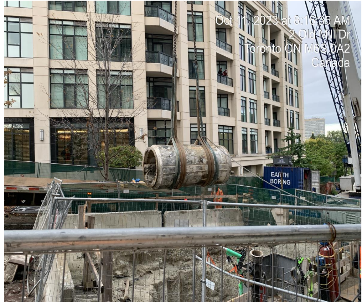
On Wednesday, October 11, 2023, MTBM's tail can retrieval operation.
