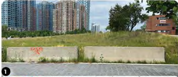
1 Constraint – Steep slope on south east of site requires retaining wall to accommodate some programs.
