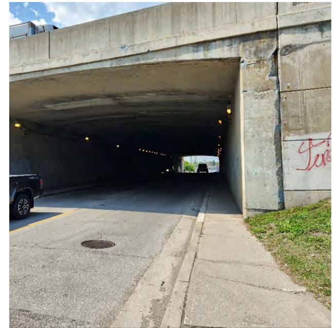
Highway 401 underpass at Wendell Avenue
