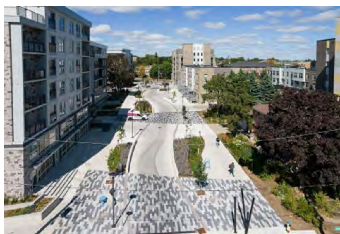
A "woonerf" in Waterloo turns quieter streets into shared spaces through traffic calming and furniture (Source: engagewr.ca)
