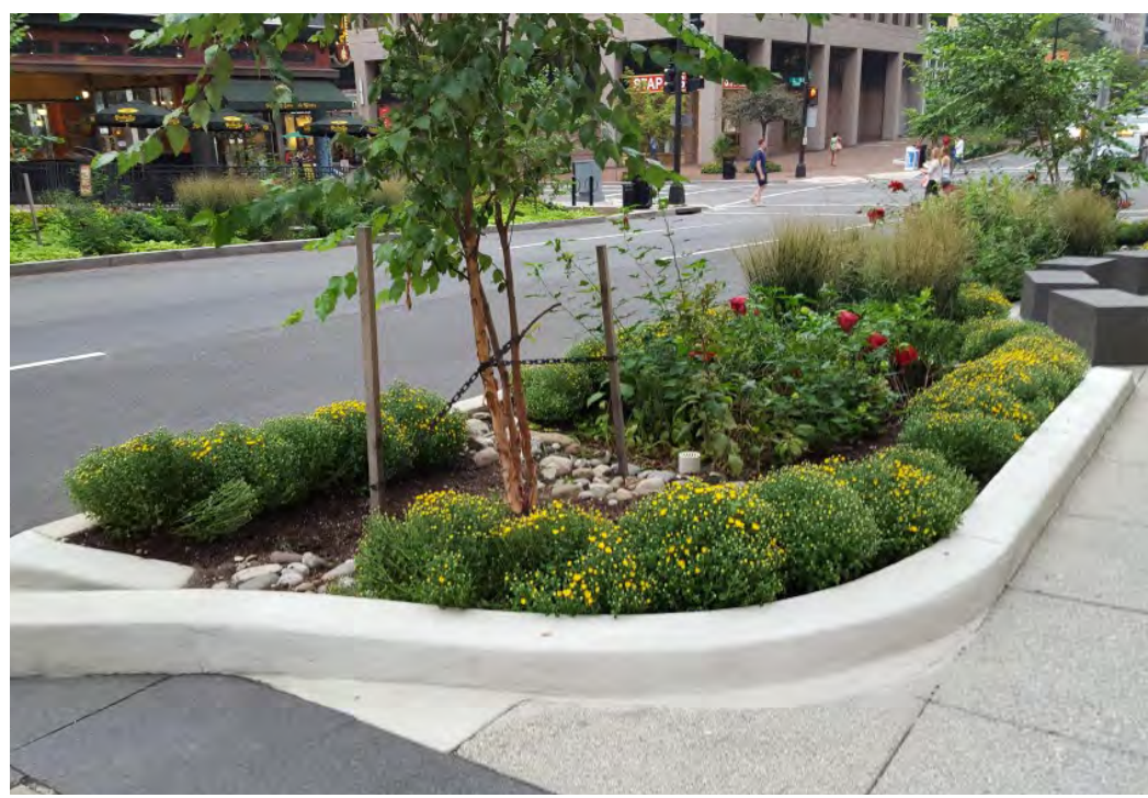
Integrating rain gardens into the streetscape can mitigate runoff and promote biodiversity within the urban landscape (Source: EPA)
