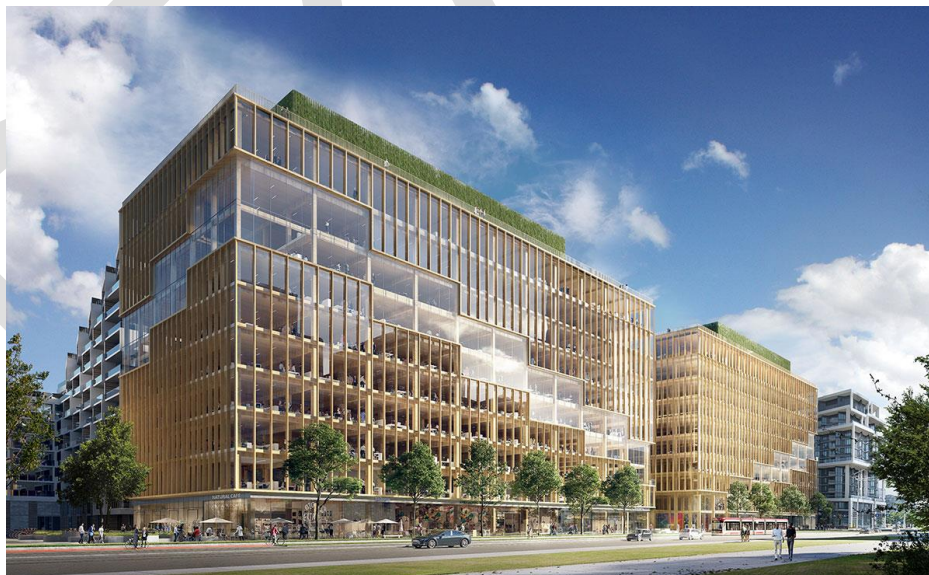
3.4 Compact built forms with fewer step-backs can be built efficiently with tall timber construction methods. T3 Bayside in Toronto is an example of architectural forms that exemplify sustainable building techniques by advancing tall timber construction.
