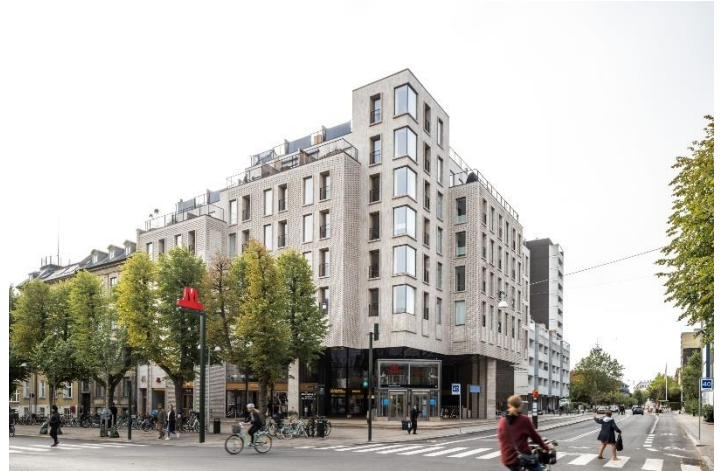
2.1 The Frederiksberg Allé development in Copenhagen, Denmark incorporates built form step-backs to reduce downdraft conditions.
