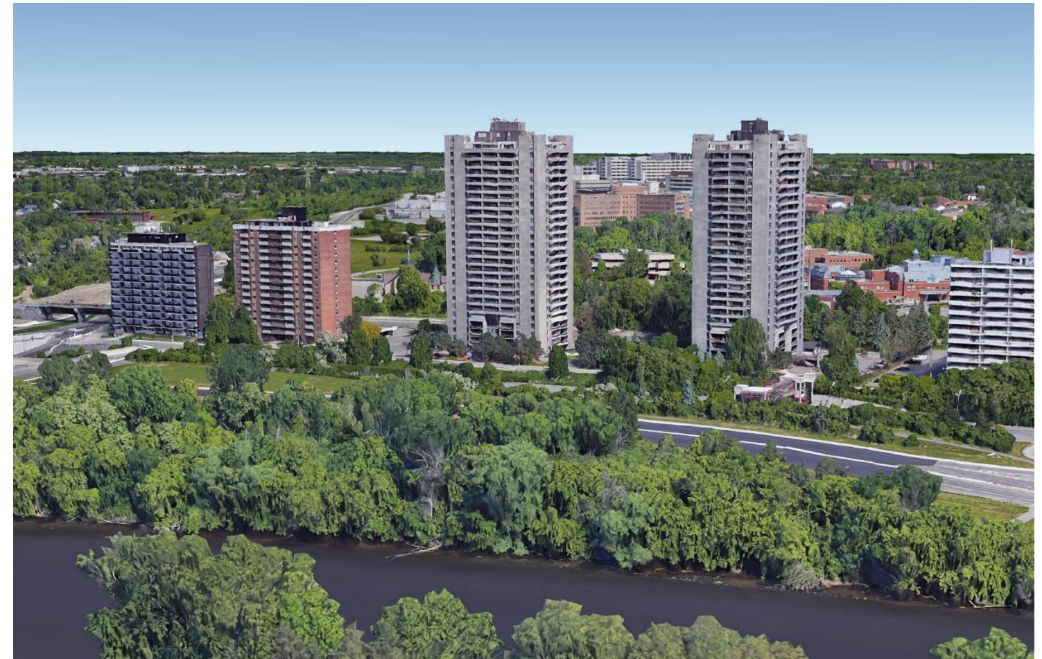
IMAGE OF 1755 FROBISHER LANE (MIDDLE) FROM GOOGLE EARTH
