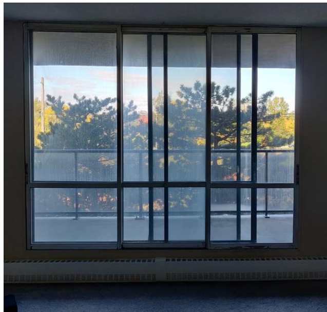
IMAGE OF SUITE WINDOW AND BALCONY FROM RDH SITE VISIT
