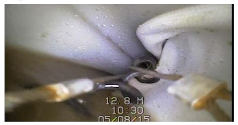
Root Cause: "Sleeving" across bend due to a greater than 45-degree bend.
