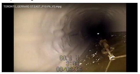
**Root Cause:** Tightly bonded cement or hard tuberculation that is resistant to pressure flushers and scrappers. Increase in number of passes or even pressure could lead to host pipe being subjected to blow holes.
