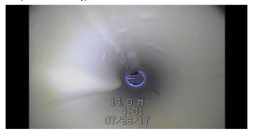
**Root Cause:** Different than standard lumps, its shape is caused by instantaneous depressurization or rapidly pushed up air during lining due to an adjacent valve.
