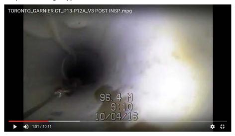
Root Cause: Lining over an existing substandard service that has not been grinded down.
