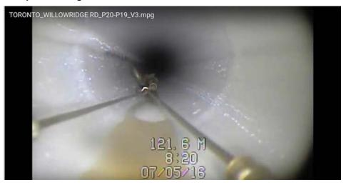
**Root Cause:** Bump due to external pressure (water or air) during the forming of the liner. **Description:** Small size ovoid lump along the bottom of the liner. Width at the lump base is <10% of the circumference of the liner. Height of the lump is <10% of the diameter of the liner. Lump poses no problem to the liner.
