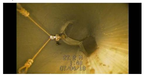
**Root Cause:** Commonly occurs when there are multiple bends in a run as well as large axial folds at the bends. The bends cause tension in the CCTV winching rope resulting in contact between the fold and the rope. This action causes tearing or fraying of the liner fold at the bends.
