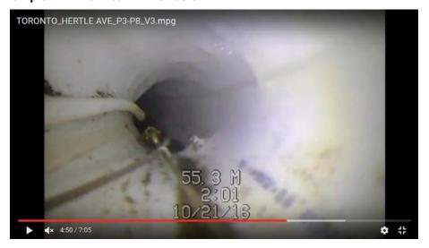
Root Cause: Abrasive action of winching mechanism while pulling CCTV camera equipment.
