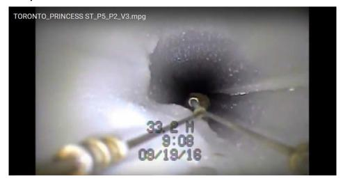
**Root Cause:** Lead deposit at the base of the pipe due to improper pouring of lead when joining pipe together. The lead could not be removed by cleaning.
