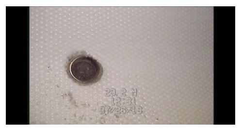
**Root Cause:** Epoxy plugged services due to missed or incorrectly installed plugs. **Description:** Migration of epoxy into the service line rendering the water service inoperable.
