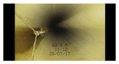
Root Cause: Liner collapse caused by mater meter being turned on at adjacent home with service open.
