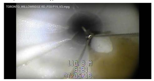
Root Cause: Bump due to external pressure (water or air) during the forming of the liner.
