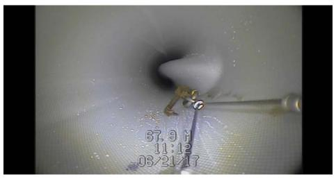
**Root Cause:** This section was below two water services, assumption is that there was a leak overnight through the lining day which accumulated water at the base of this section and was then lined over.
