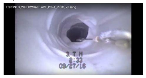
Root Cause: "Accordion" effect due to accumulation of material during the forming stages.
