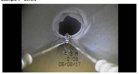
**Root Cause:** "Accordion" effect due to accumulation of material during the forming stages. Liner not property stretched out after being threaded through host pipe
