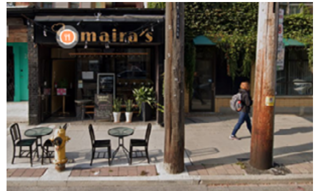
Distribution/Street Lighting Pole
