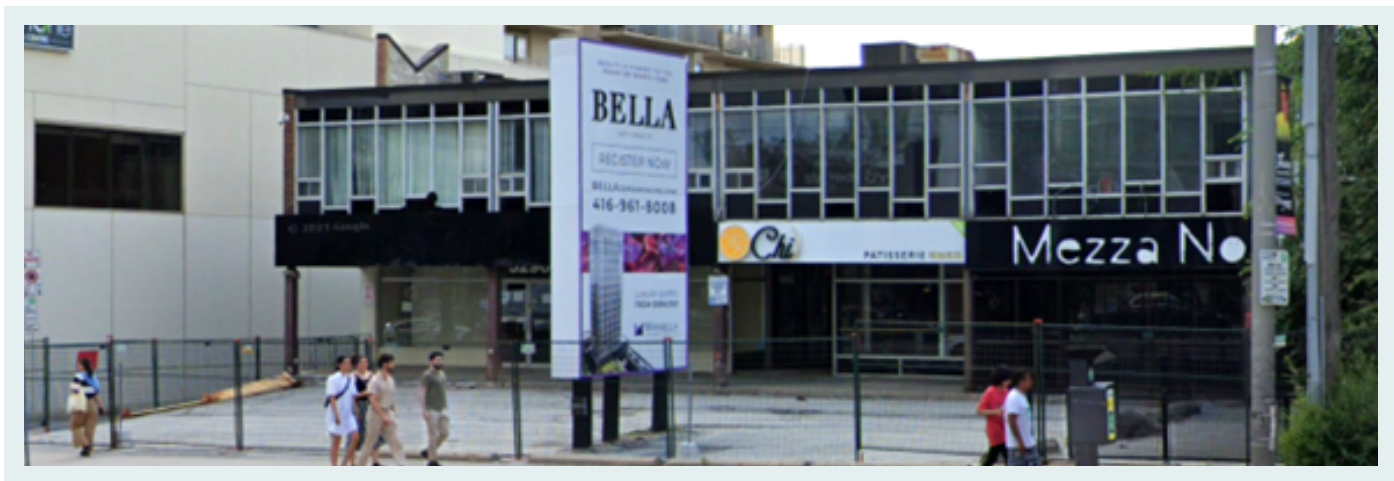
Figure 24 - Former Strip Plaza at 5300 Yonge Street Fenced Off for Redevelopment (Source: Google Images)
