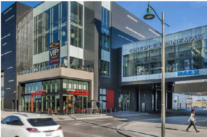
Figure 212. Through consultation, many youth wanted to see a movie theatre in the neighbourhood. This example is from Markham - anchor uses like a Cineplex and York University are integrated into development (Downtown Markham)
