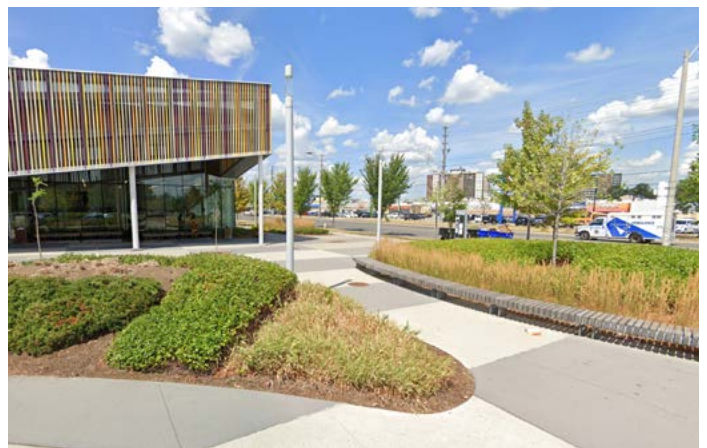
Figure 199. Paving, landscaping, and canopies provide comfortable spaces at-grade - Albion Library, Toronto (Google Maps)
