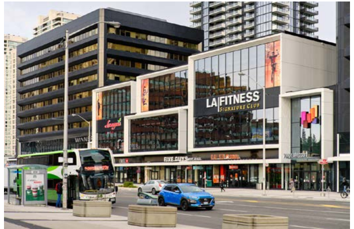
Figure 216. Yonge-Sheppard Centre features taller storey heights to accommodate non-residential uses such as supermarkets, restaurants, gyms, and retail (Archilovers)
