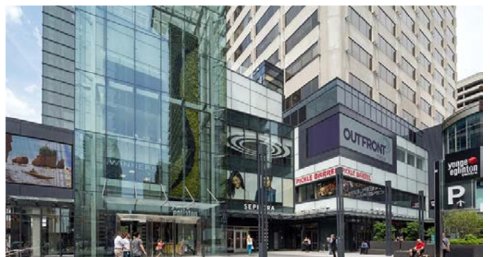
Figure 218. Ground floors - lobbies, retail shops, restaurants, should promote visibility and transparency - Yonge Eglinton Centre, Toronto
