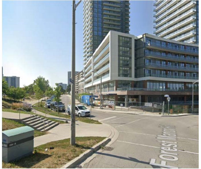
Figure 220. Towers and base buildings should be shaped, located, and oriented to preserve comfortable conditions for pedestrians, with consideration for microclimate (wind and sun) – Forest Manor Road, Toronto
