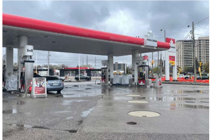
Figure 209. Gas station at southwest corner of Jane and Finch (Perkins&Will)
