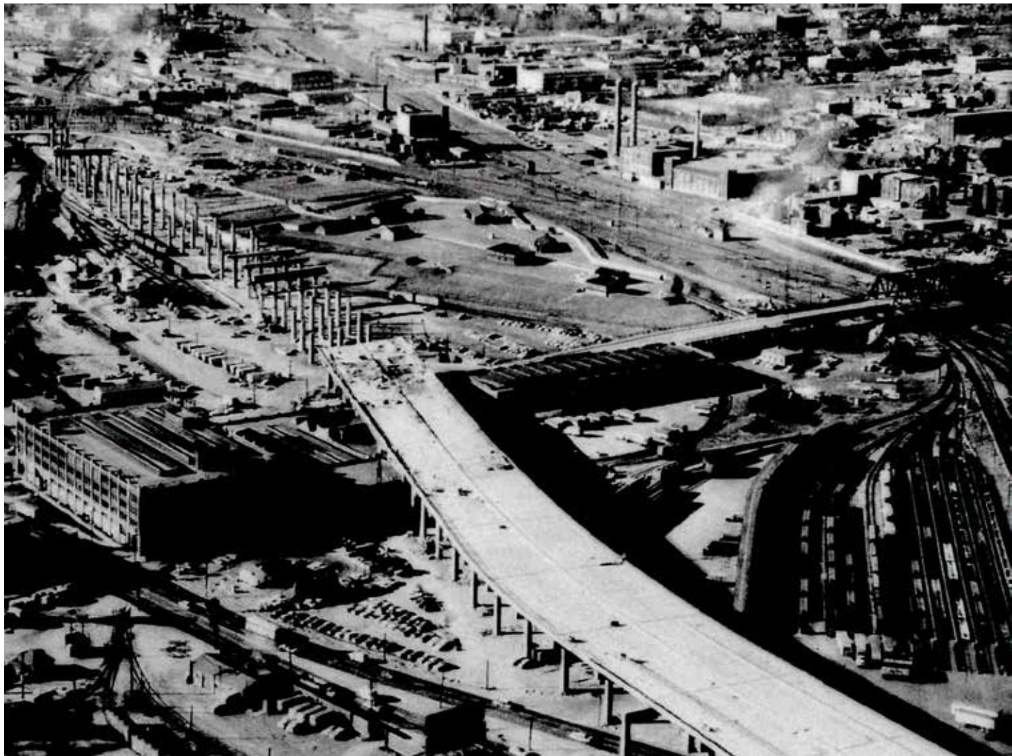
1960s, Construction of the Gardiner Expressway
