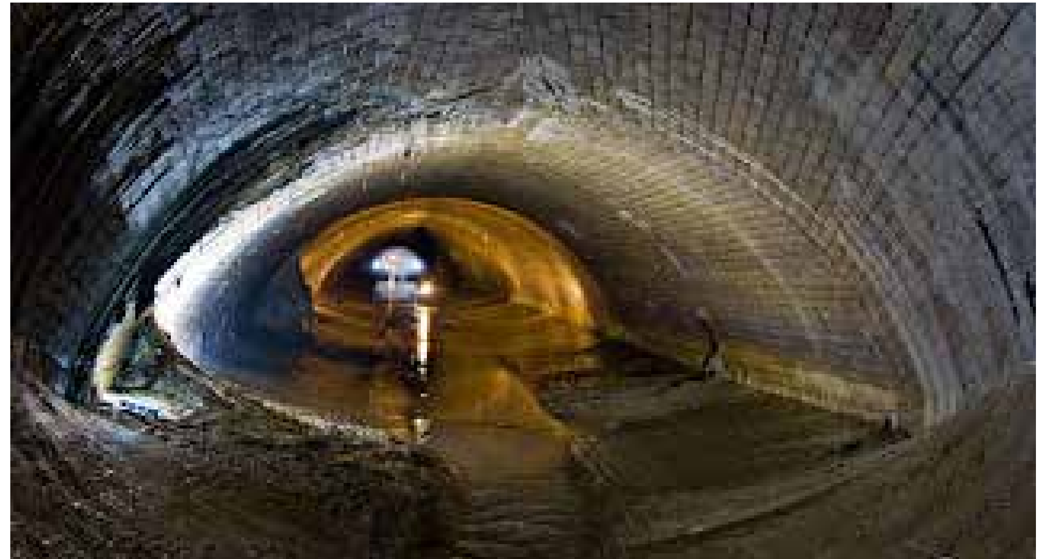
2010, Garrison Creek Sewer
