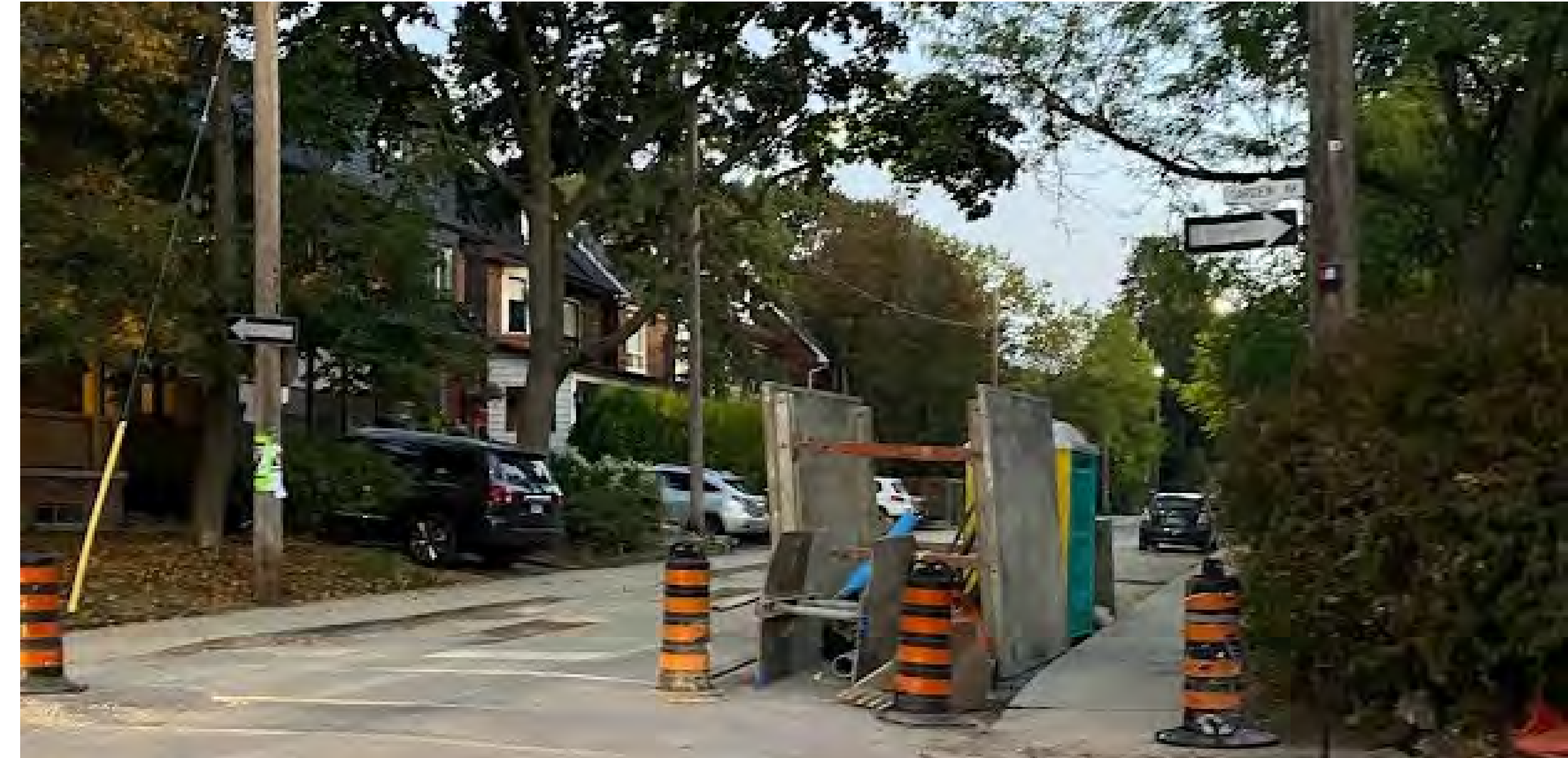
Watermain rehabilitation in the neighbourhood
