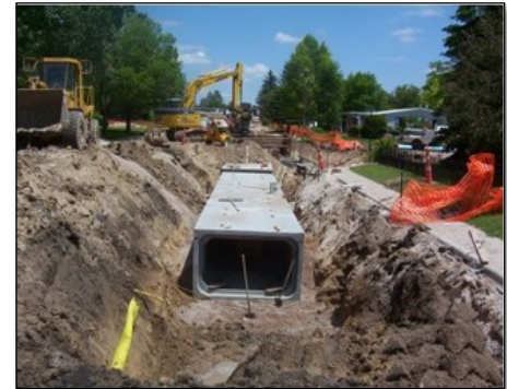
An illustration of a box culvert
