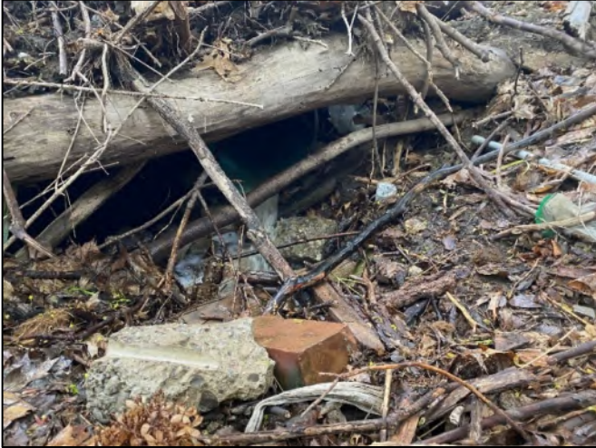
Photo 1: Site 58-28, main storm outfall
