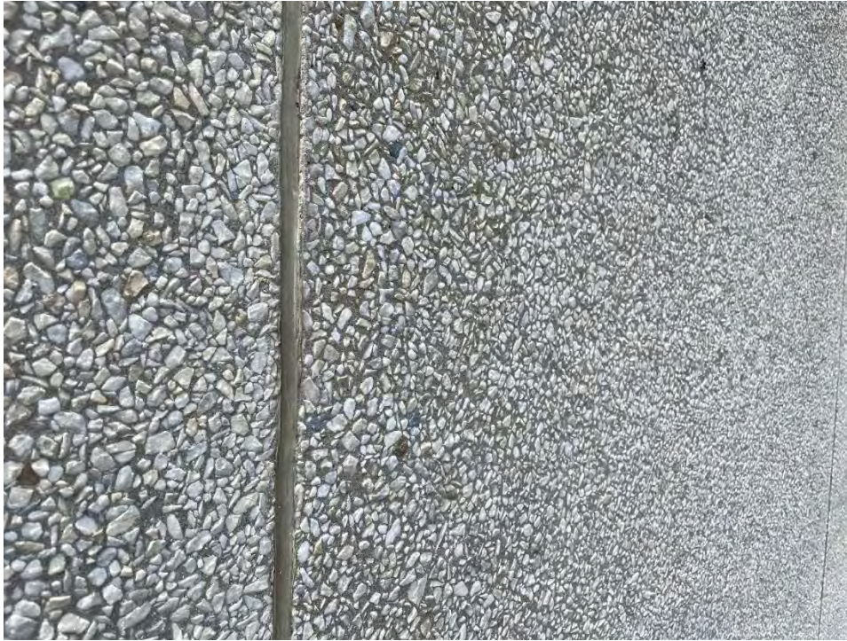
Figure 21: Typical concrete cladding with exposed aggregate.
