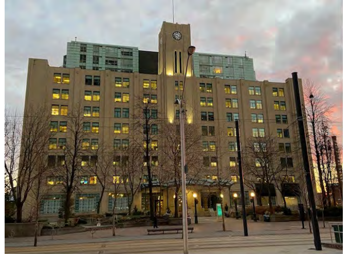
Plate 8: View of the Terminal Building, facing south.
