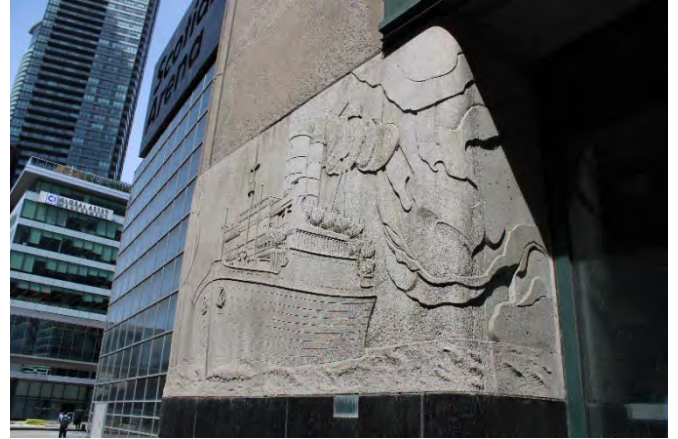
Plate 22: View of bas relief sculpture on the south elevation of structure. Note that this sculpture marks the point along the south elevation where the original façade ends.
