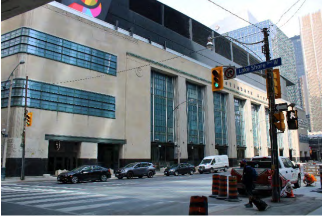
Plate 17: View of the east elevation of 40 Bay Street, looking northwest.
