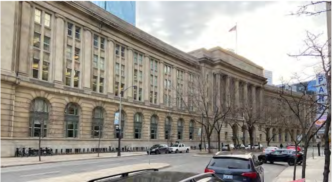
Plate 6: View of the Dominion Public Building, facing southwest.
