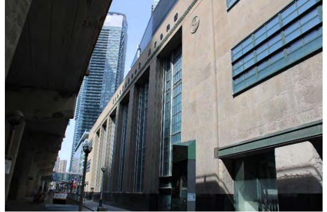
Plate 18: View of the south elevation of 40 Bay Street, facing west-northwest. Note the proximity to the Gardiner Expressway (left).
