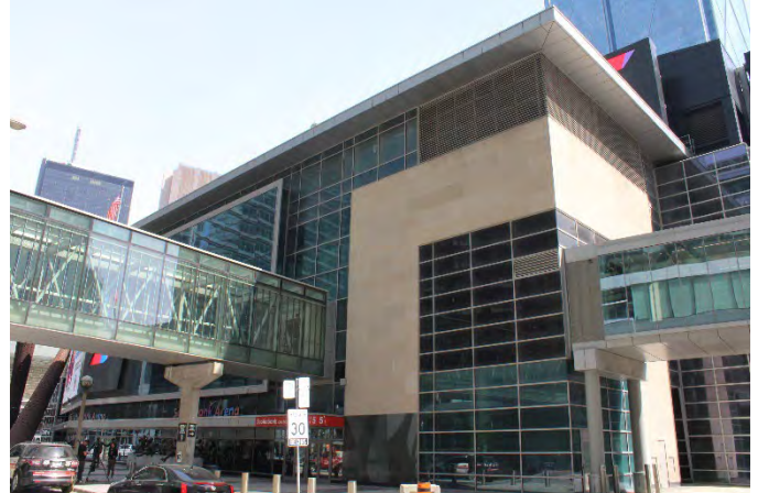
Plate 16: View of the west elevation of Scotiabank Arena showing teamways that connect infrastructure in the area to the arena, facing southwest.
