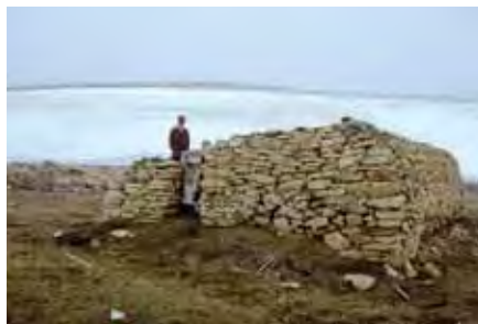
Responding to the dangers of arctic exploration and the loss of the Franklin Expedition, Kellett's Storehouse in Nunuvut was built in 1853 for sailors in distress. Constructed from local stone, it was filled with enough provisions to maintain a large group for several months. Conserving building remains or above-ground archaeological resources pose unique challenges. In this case, the walls and foundations were stabilized and an insulated floor was installed allowing remaining soil layers and associated artifacts to be left in place while being protected from theft and further exposure to the elements.
