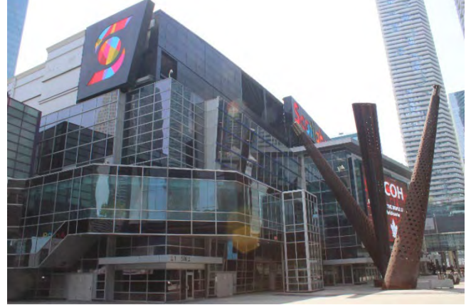
Plate 26: View of the west elevation of 40 Bay Street, facing southeast. This shows the modern irregular design, vibrant signage, and sculptural embellishment located along the west elevation.
