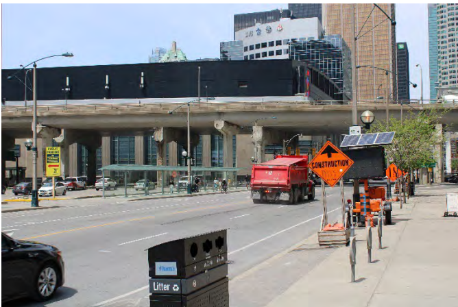
Plate 13: View of the Scotiabank Arena looking north from Bay Street. This view shows the proximity of the Gardiner Expressway to the structure.
