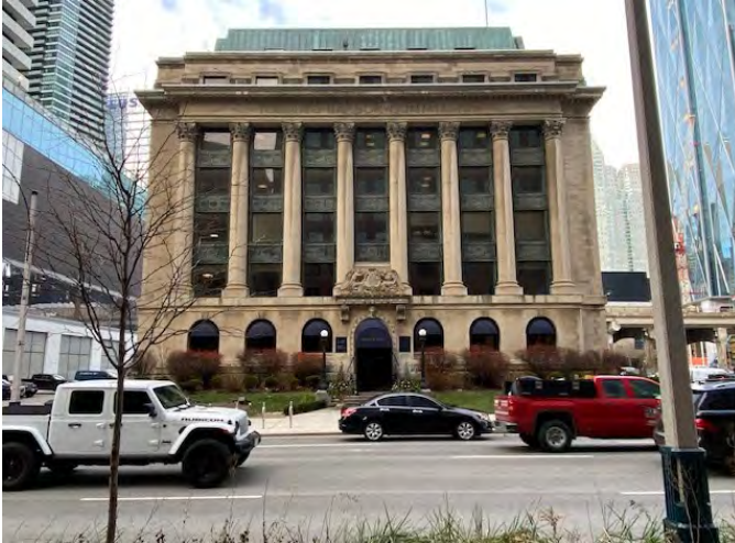
Plate 7: View of the Toronto Harbour Commission Building, facing north.
