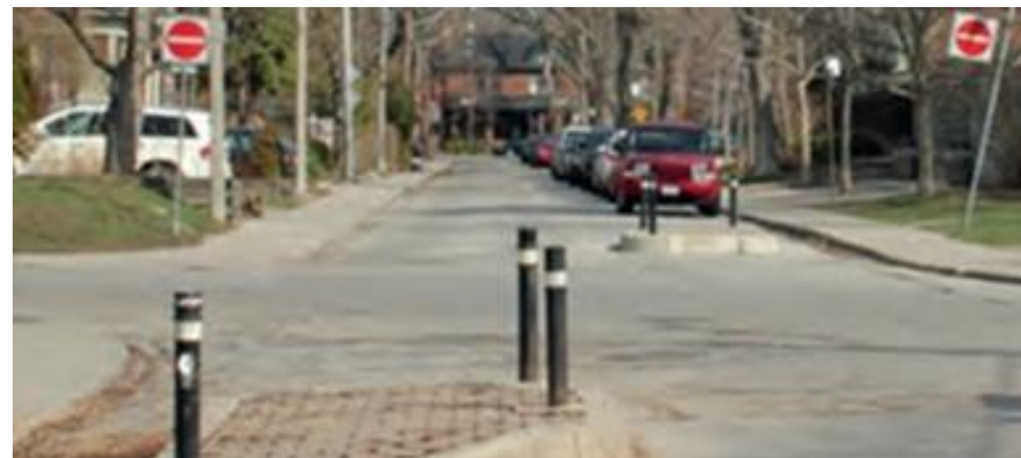
Curb extension to reinforce a directional closure
