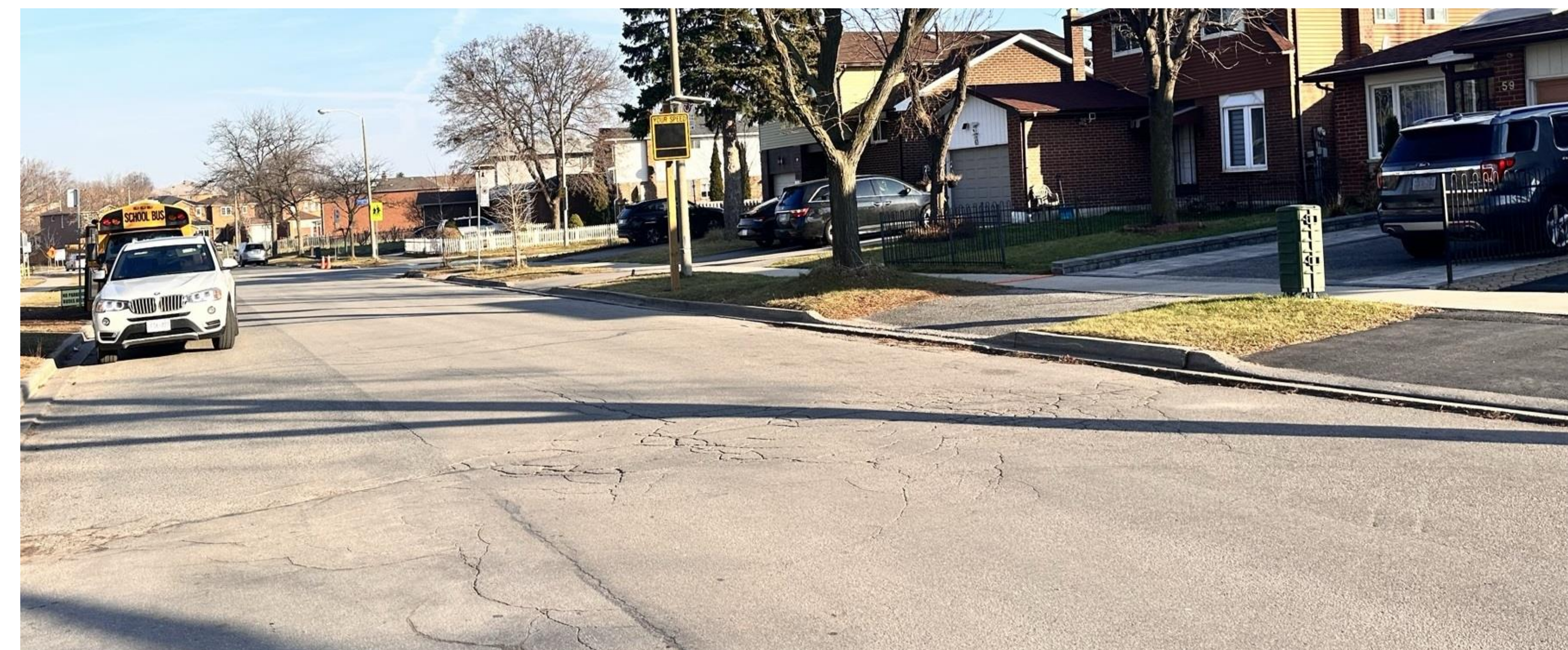
A neighbourhood street at Malvern West
