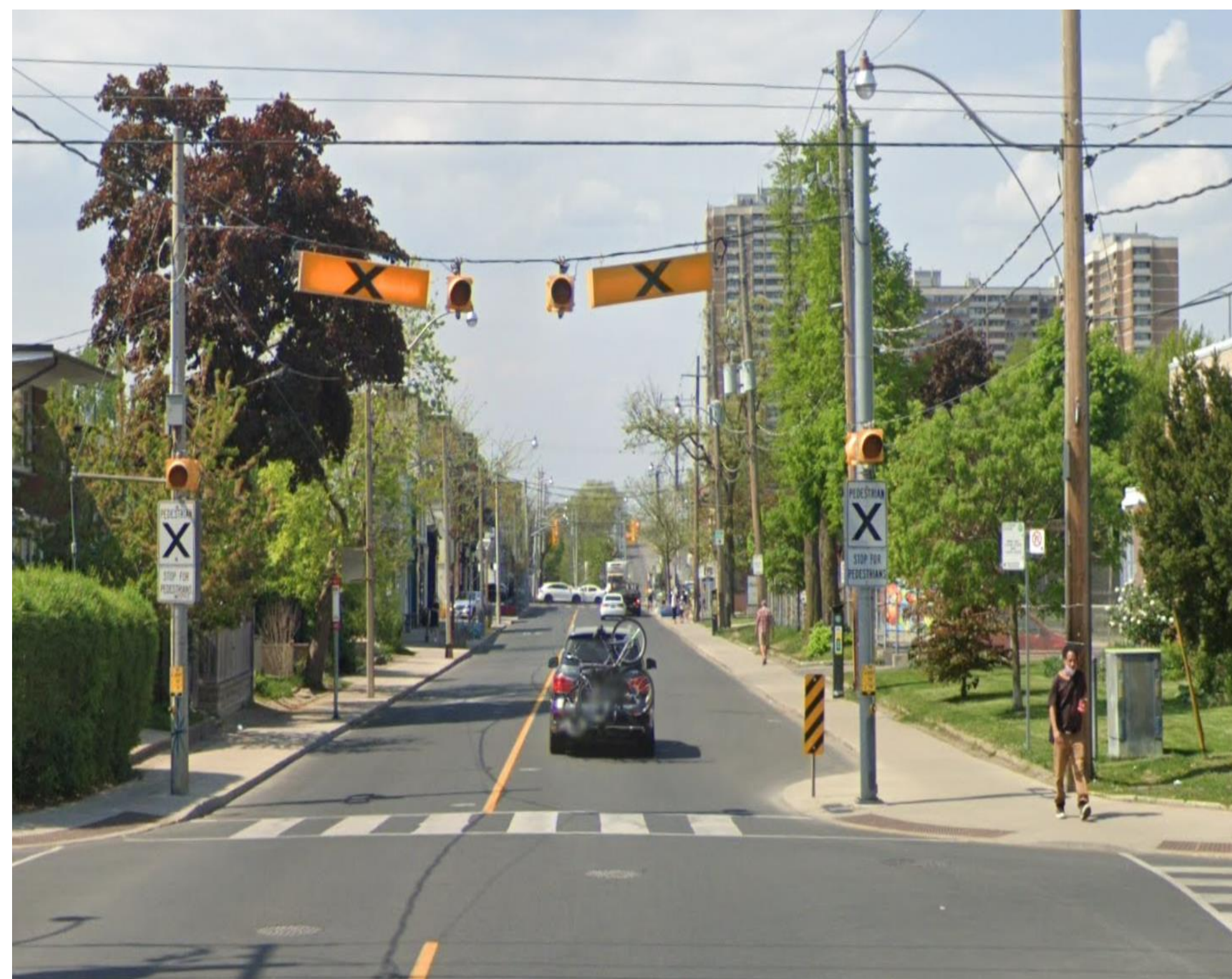
Curb extension with concrete and asphalt and signage
