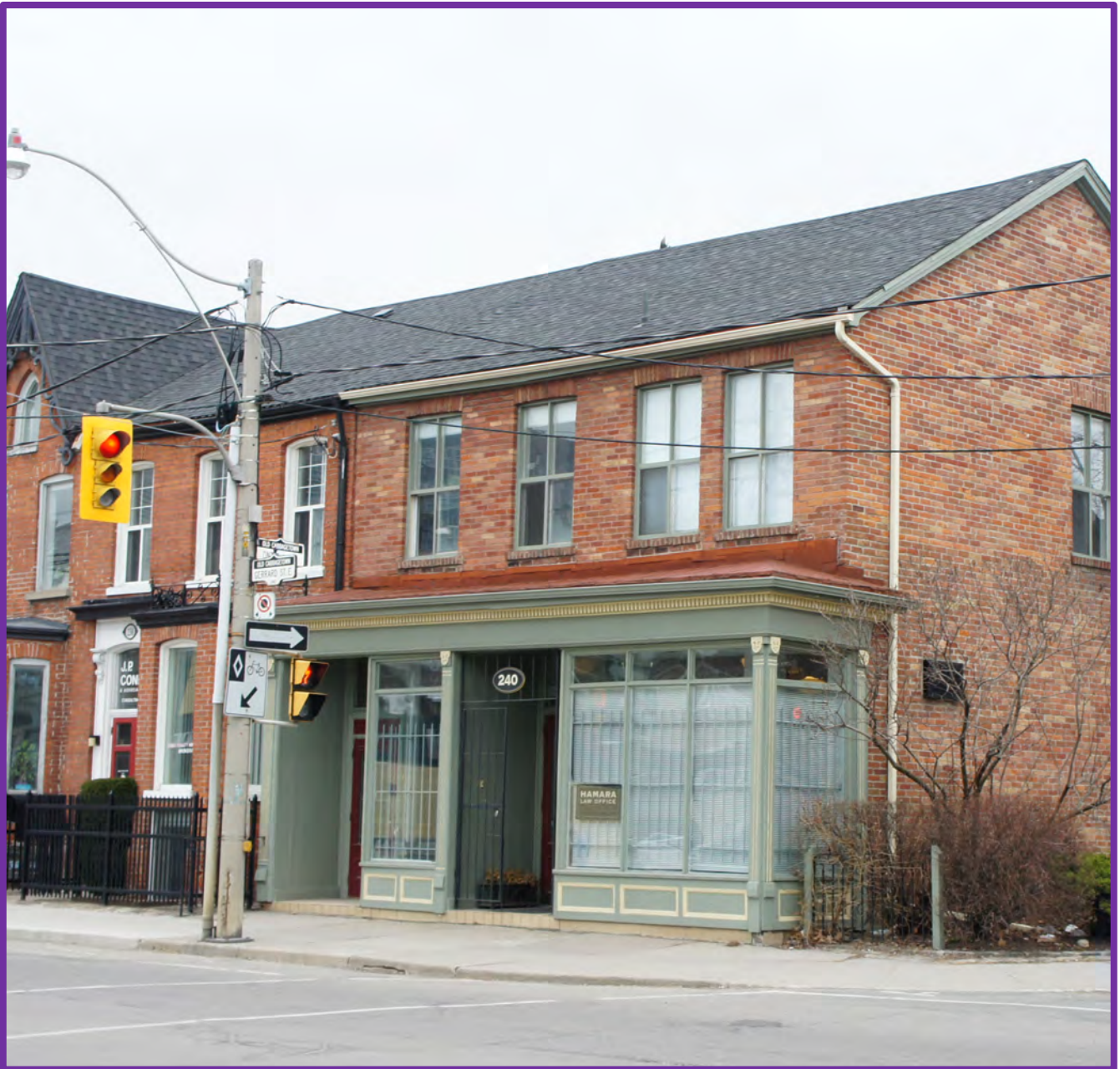
Figure 70: Historic storefront at 240 Gerrard St. E.
