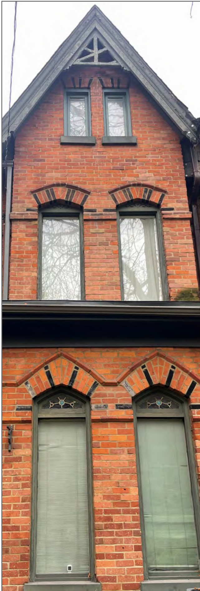
Figure 68: Retention of ground floor transoms at 175 Seaton St.
