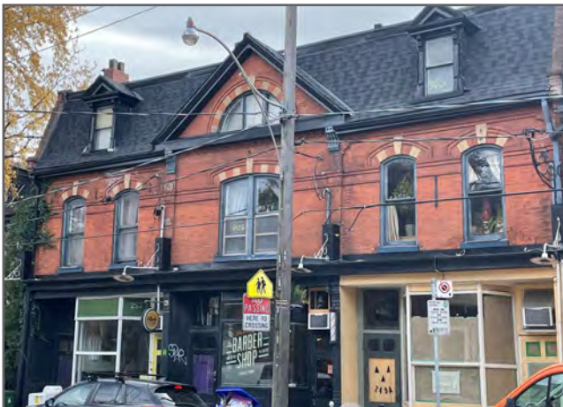
Figure 32: 249 - 253 Gerrard St. E.
