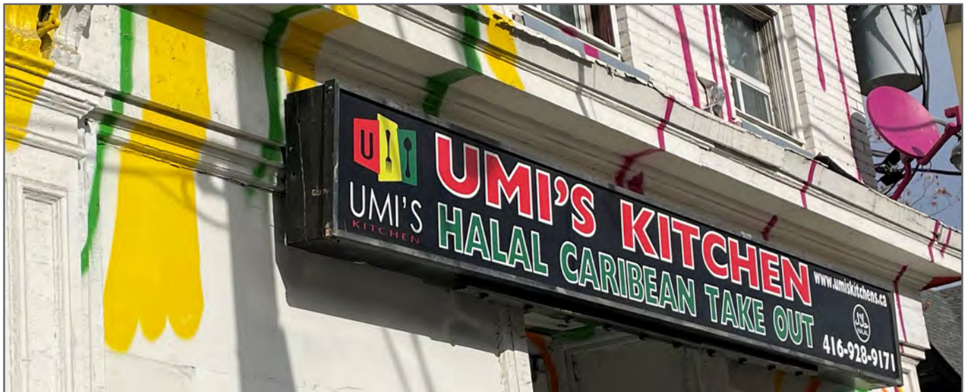
Figure 75: Existing signage on historic storefront at 346 Dundas St. E.; existing fascia boards (sign bands) should be utilized for contemporary signage.
