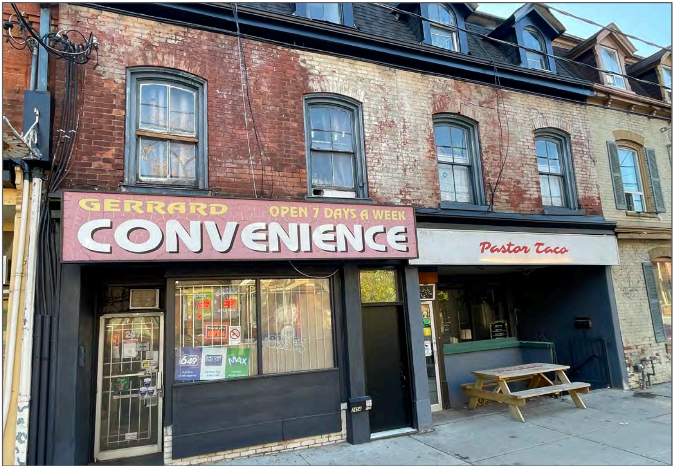
Figure 72: Gerrard St. E. storefront with non-historic finishes.
