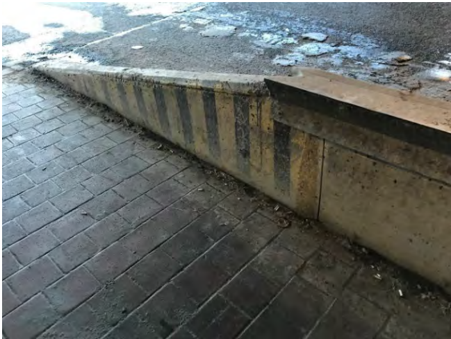
Plate 24: View of the concrete partition and brick walking surface at the north end of the west teamway in the Bay Street underpass.
