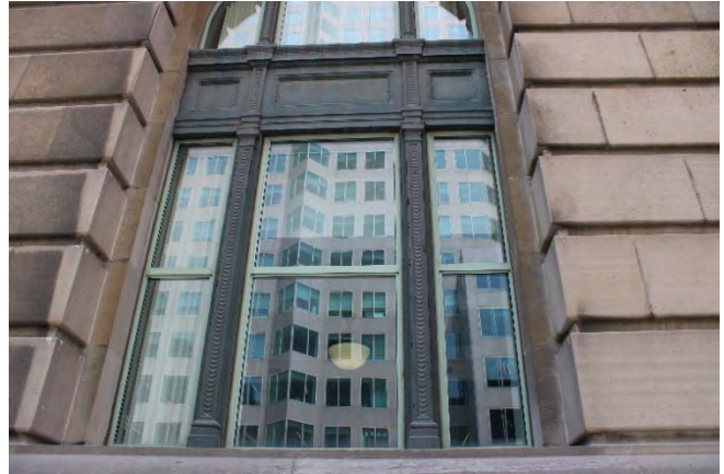
Plate 51: Example of a first-storey window on the west elevation featuring metal mullions incorporating rope detailing
