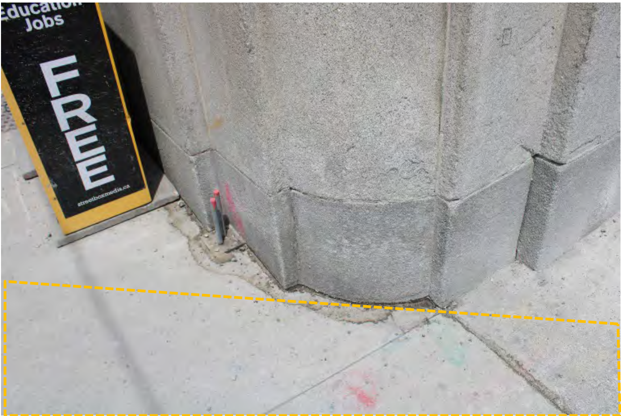
Plate 61: Southwest corner of the Dominion Public Building at curb connection with a rounded corner with vertical clean cut detail. A new, below-grade wall will be constructed that will abut this corner of the building.
