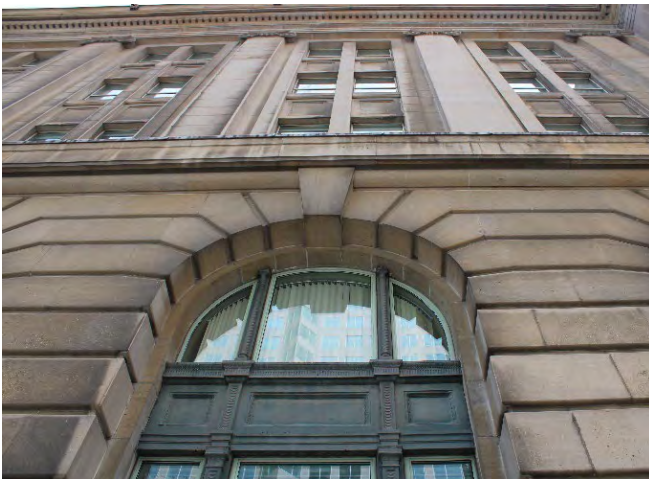
Plate 52: Example of a first-storey window on the west elevation featuring metal mullions incorporating rope detailing
