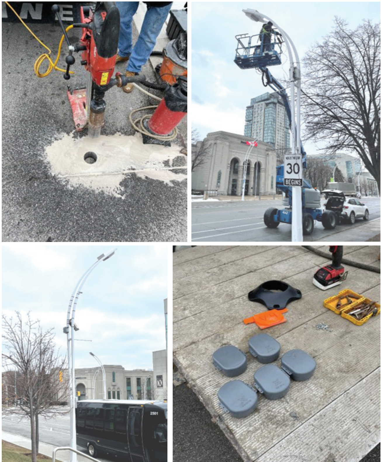
Figure 3: Clockwise from top left: Coring for the Electromega installation, Automotus camera installation in progress, eleven-x sensors prior to installation, Precise ParkLink (Mistall) post installation
