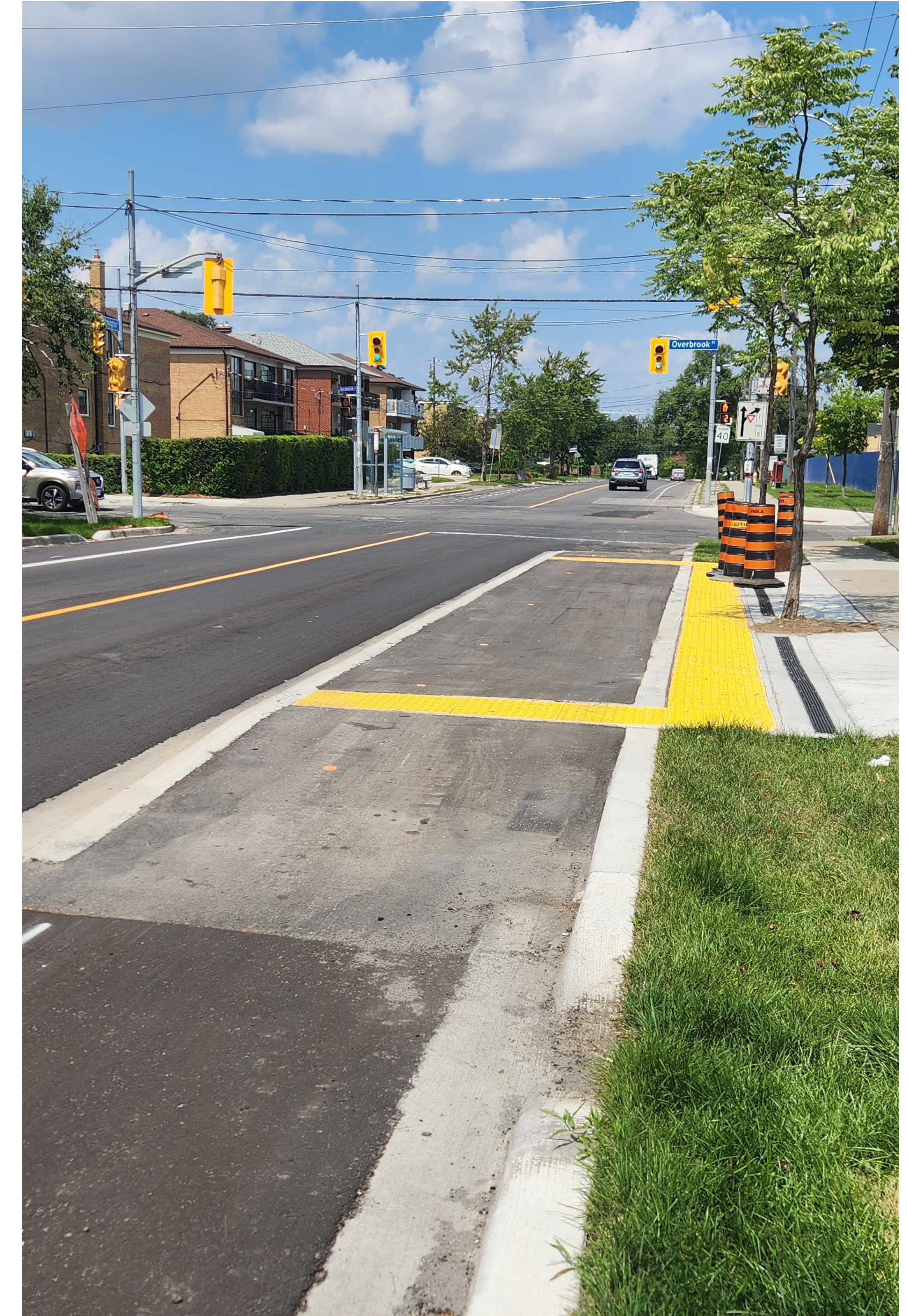
Raised bus and bike transit stop on Wilmington Avenue
