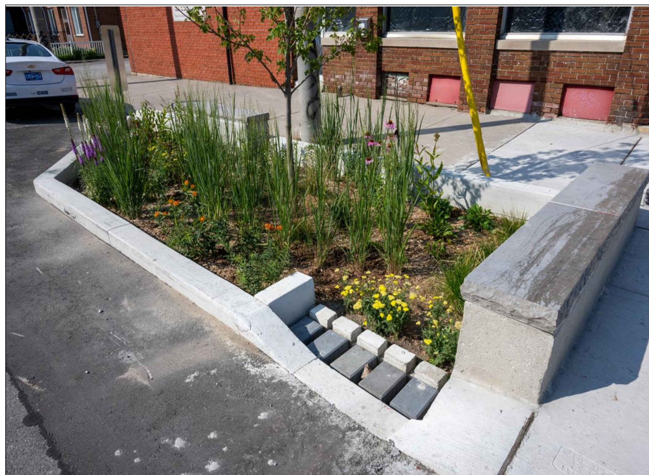
Curb extension with concrete and asphalt
