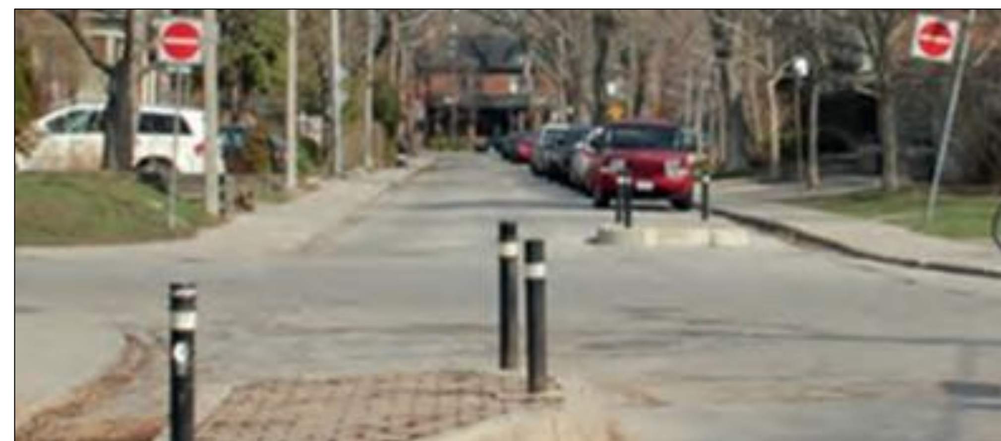
Curb extension to reinforce a directional closure
