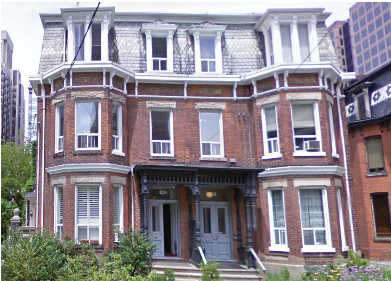
Image 2. 62-64 Charles Street East. Front (south) elevation. June 2013. Photo by John Doe.
