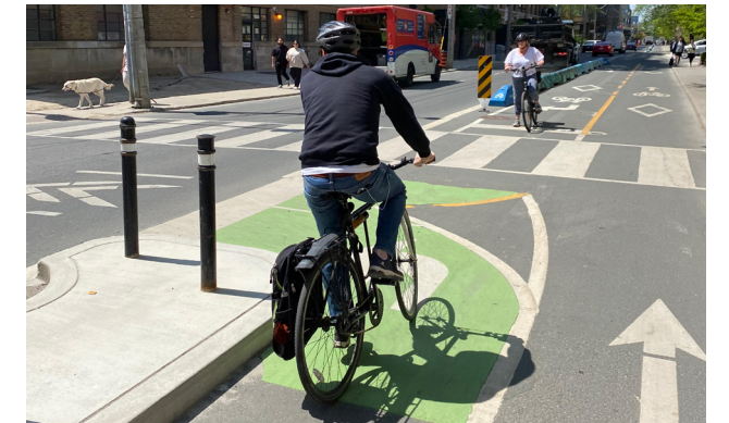
Upgrading existing intersections for safety and comfort by adding protected features such as poured-in-place concrete medians, corner islands or reducing curb radii.
