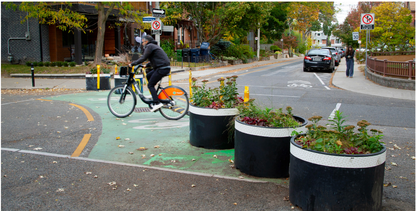
Image 1. A diagonal diverter is located at the intersection of Lindsey Avenue and Gladstone Avenue, which forces drivers to turn either westbound or eastbound, while people cycling and pedestrians are permitted to travel in all directions. Photo by Elsa Hashemi.
