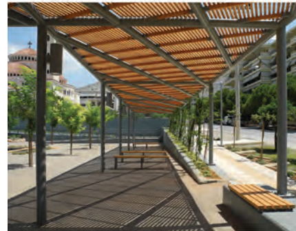
Shade structures & canopy
