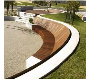
Retaining wall bench
