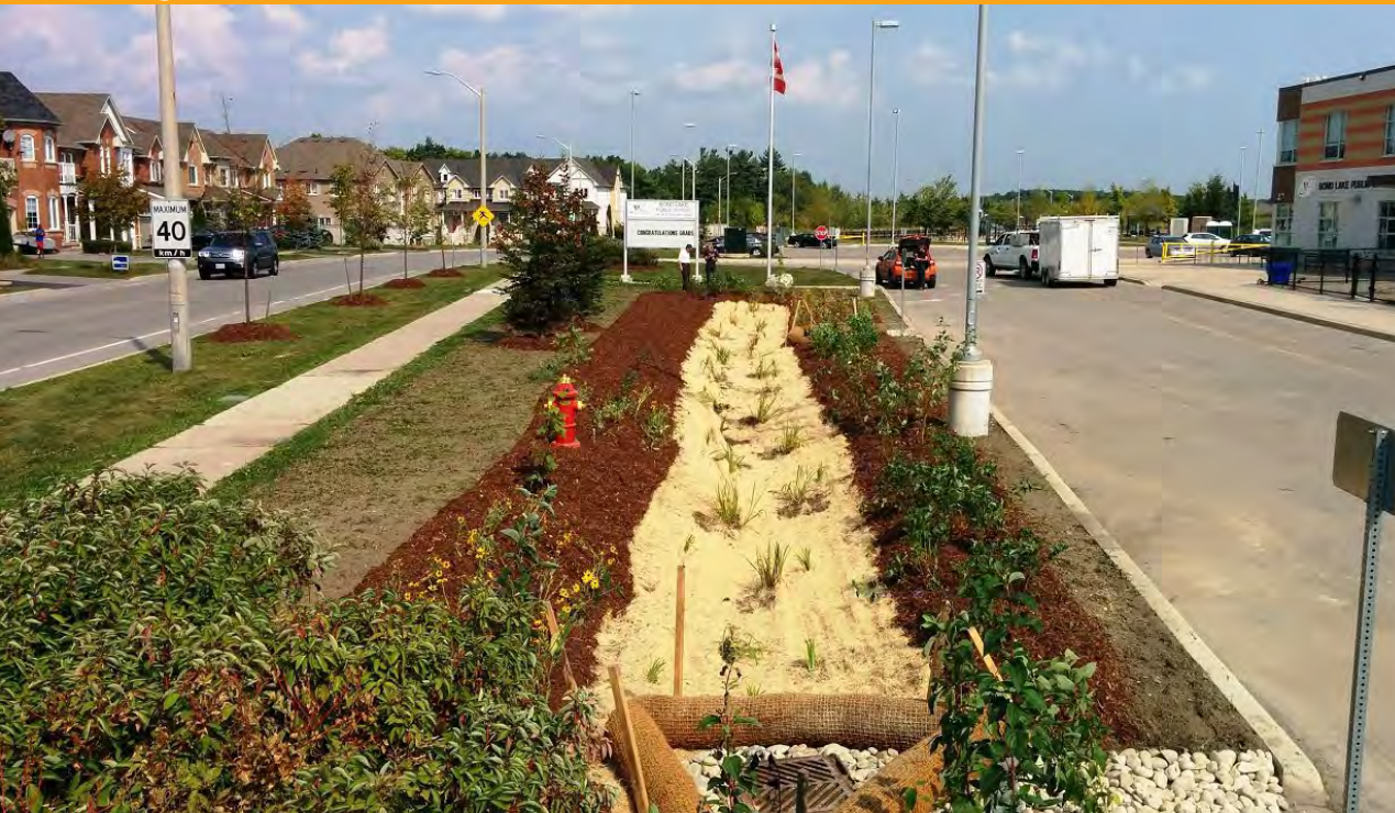
Freshly installed bioswales
