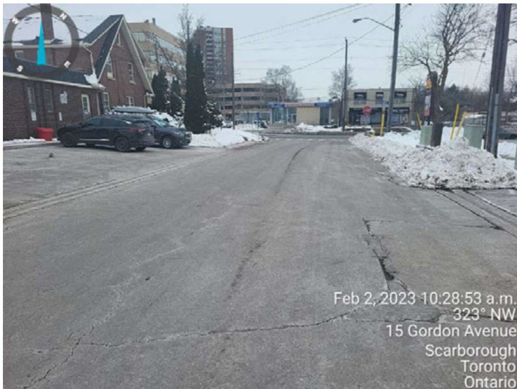
Photograph 8 – Severe joint opening and pop-outs around old patch repair. Meandering cracking on pavement surface.
