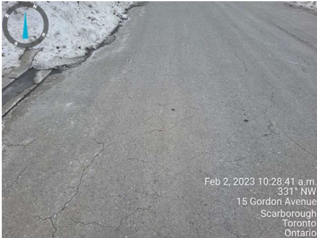
Photograph 7 – Moderate severity random/alligator cracking throughout pavement as noted in close up.
