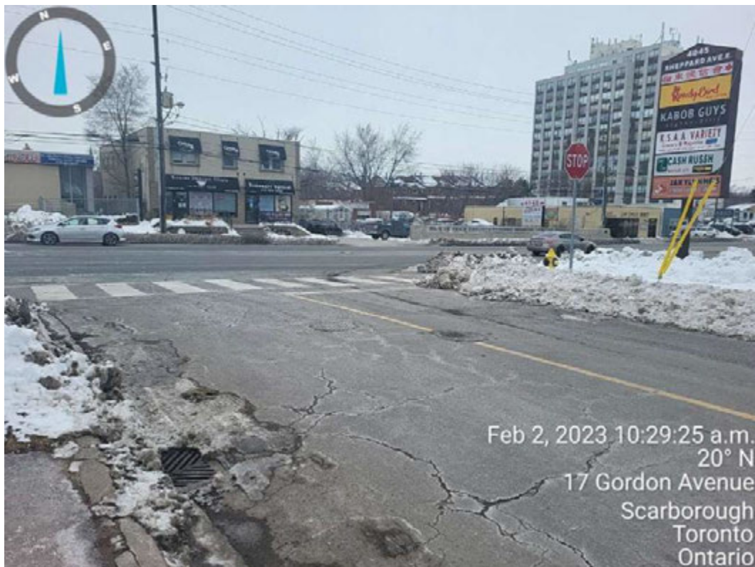
Photograph 10 – High severity localized alligator cracking around utilities. Intersection with Sheppard Avenue East.
