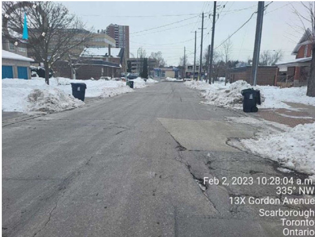
Photograph 5 – Severe cracking, disintegration and potholes in Northbound Lane.
