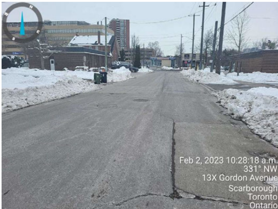
Photograph 6 – Severe joint opening and localized cracking around old patch repair. Localized cracking around utilities also visible.
