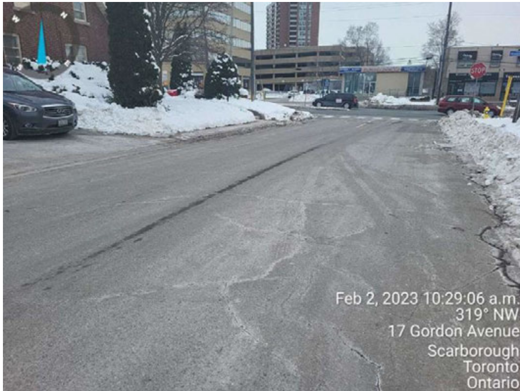
Photograph 9 – Moderate severity meandering cracking.
