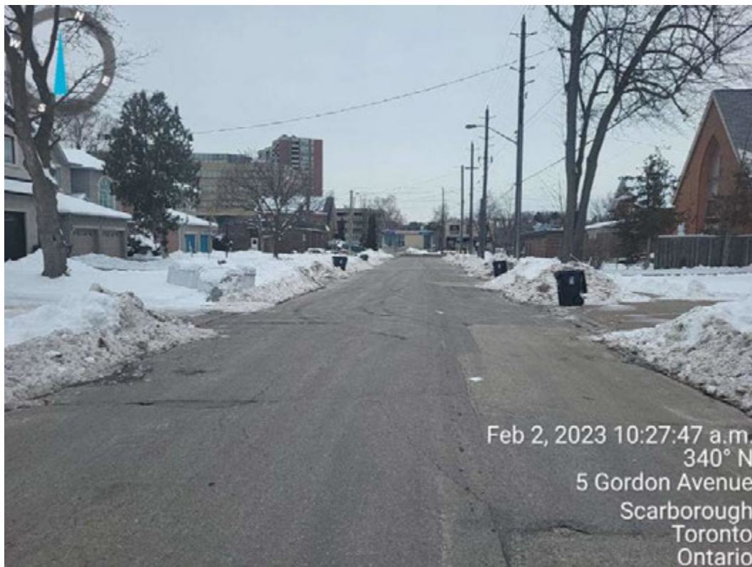
Photograph 4 – Medium severity transverse cracking. Old patch repair with joint openings visible. Pothole in Southbound lane patched.
