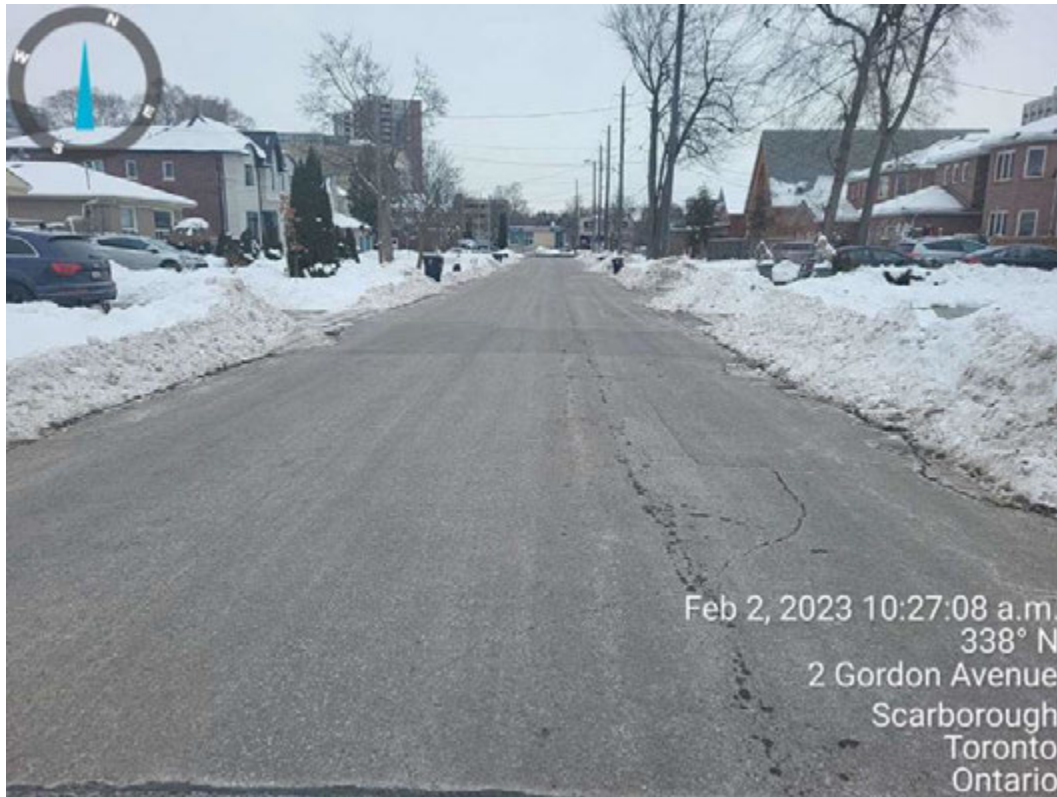
Photograph 3 – Meandering cracking, stemming from old patch repair. Pavement in overall fair condition.
