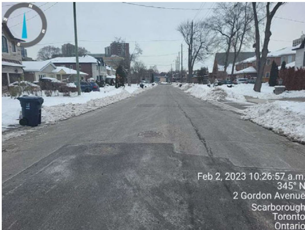
Photograph 2 – Old patch repair and crack sealing, still in fair condition. Some medium severity pavement edge cracking noted.
