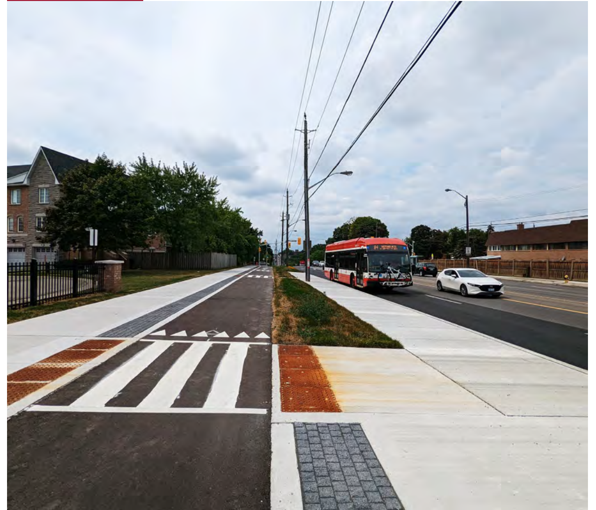
Example of Complete Street elements in Toronto.
