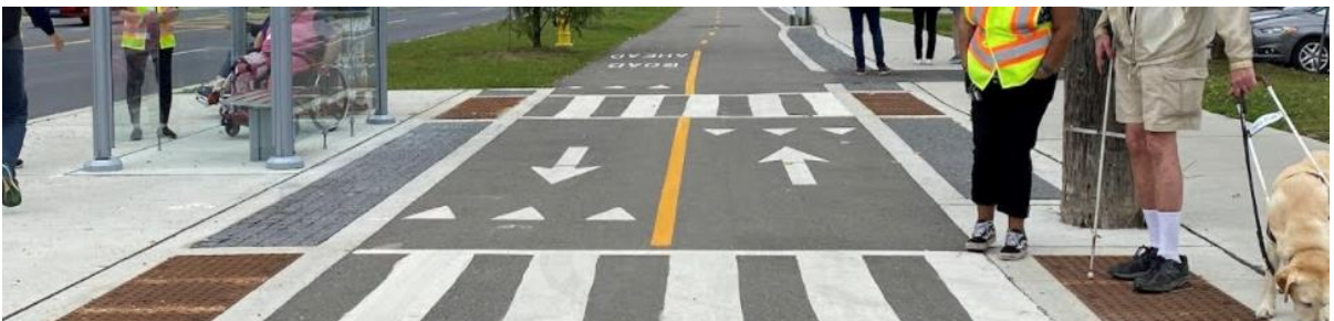
KIPLING AVENUE, NORTH OF ROWNTREE ROAD
