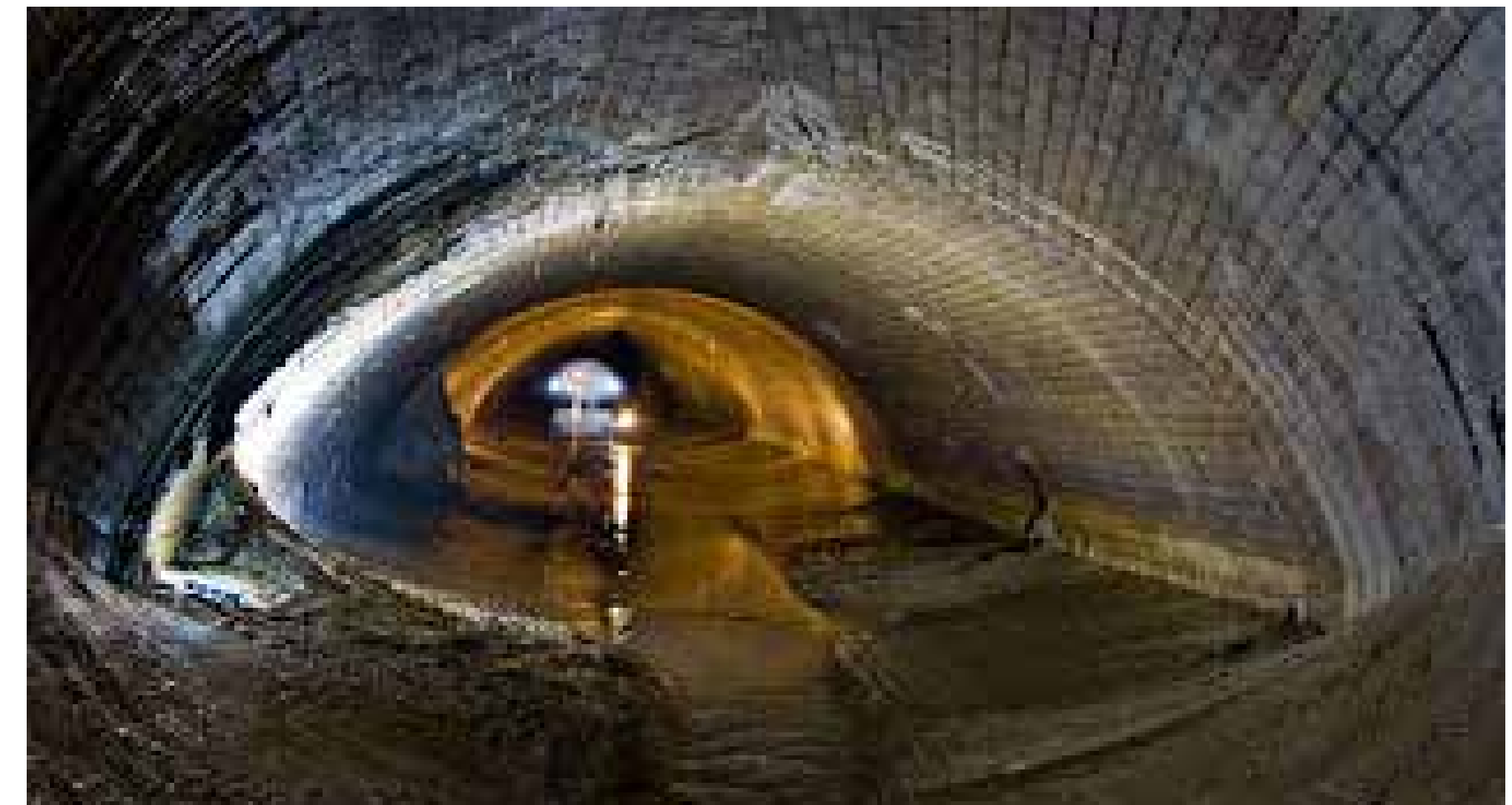
2010, Garrison Creek Sewer
