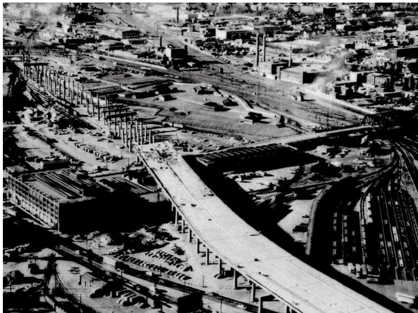
1960s, Construction of the Gardiner Expressway
