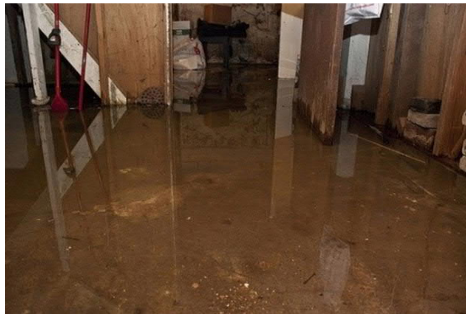
Basement flooding due to sewer overflow
