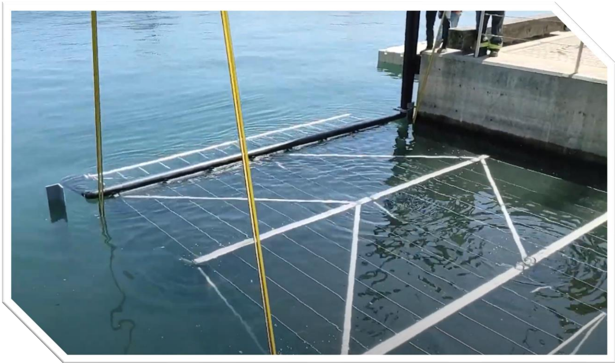
Figure 5 :Heat exchanger being lowered into Lake Ontario
