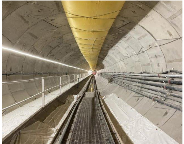
Picture of main storm sewer tunnel in construction (December 2023)
