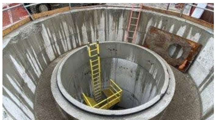
Picture of a maintenance hole in construction after micro-tunneling (October 2023)
