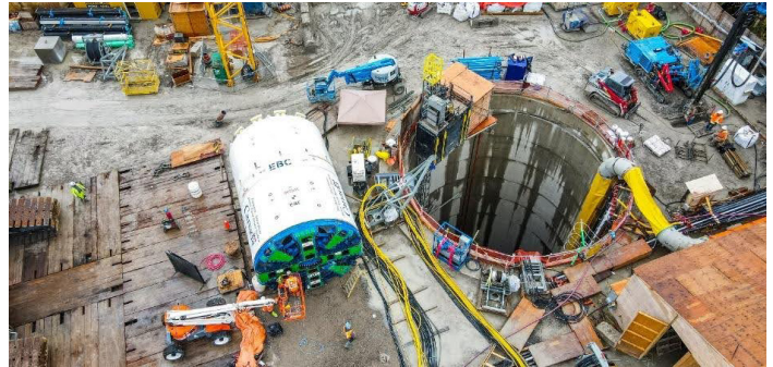
Tunnel boring machine prior to launch from the Fairbank Memorial Park (May 2023)
