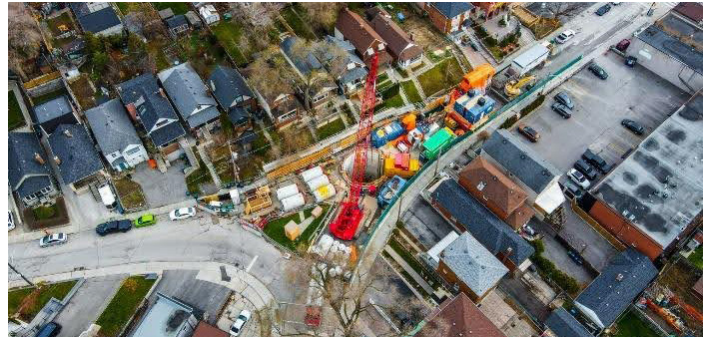
A micro-tunneling shaft during construction (September 2022)
