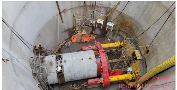
Photo of sewer pipe pushed behind the micro-tunneling machine (June 2023)
