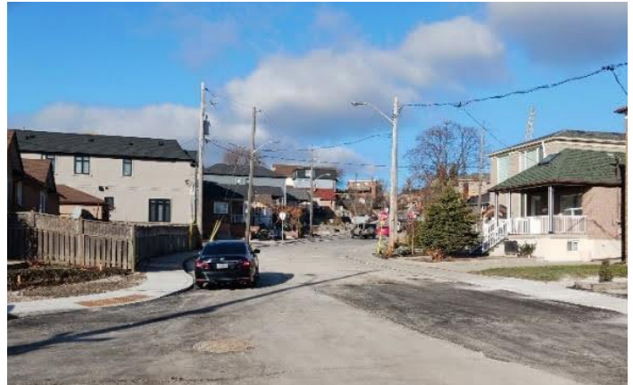
2 Chudleigh Road restored after maintenance hole completion (December 2023)
