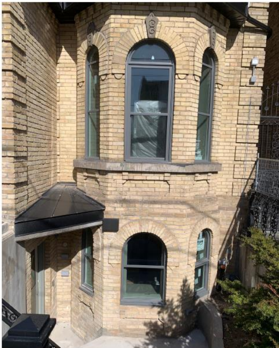
218 Carlton, Basement and Ground Floor windows
