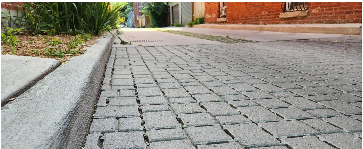
PERMEABLE UNIT PAVERS (ECO-OPTILOC)
