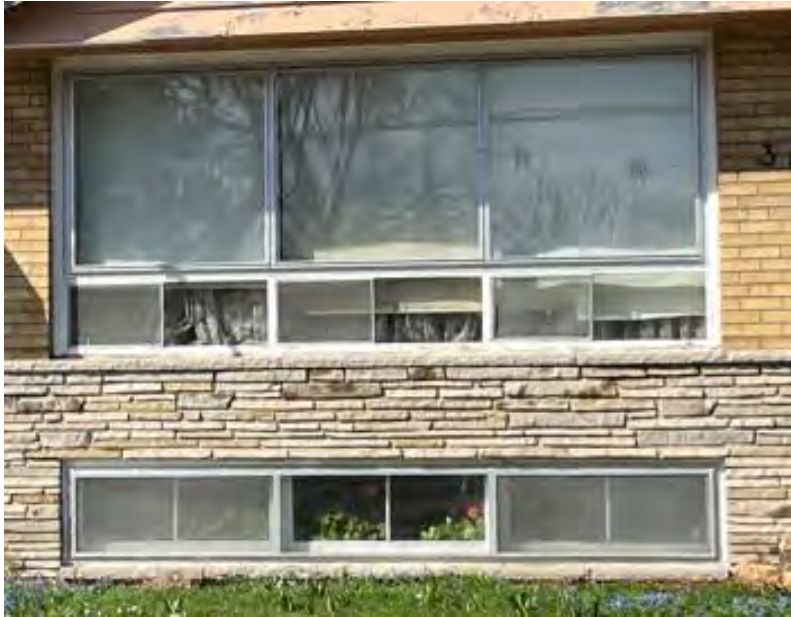
Figure 16: Detail view of the fenestration, buff brick and angel brick facing on front façade (A.S.I., 2024).
