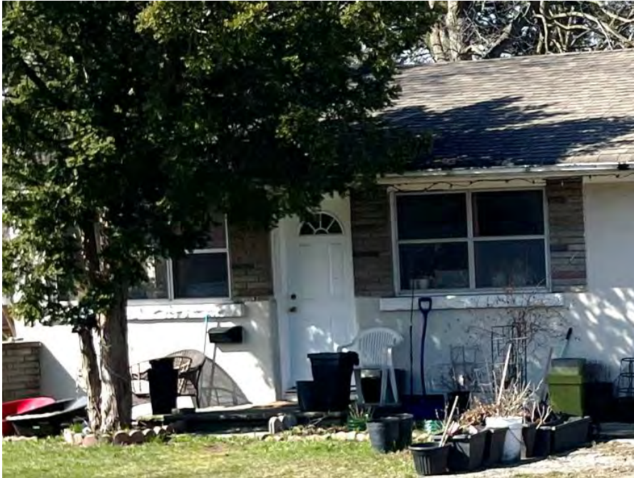
Figure 13: Detail view of stucco and brick on front façade. The concrete window sills are also visible (A.S.I., 2024).
