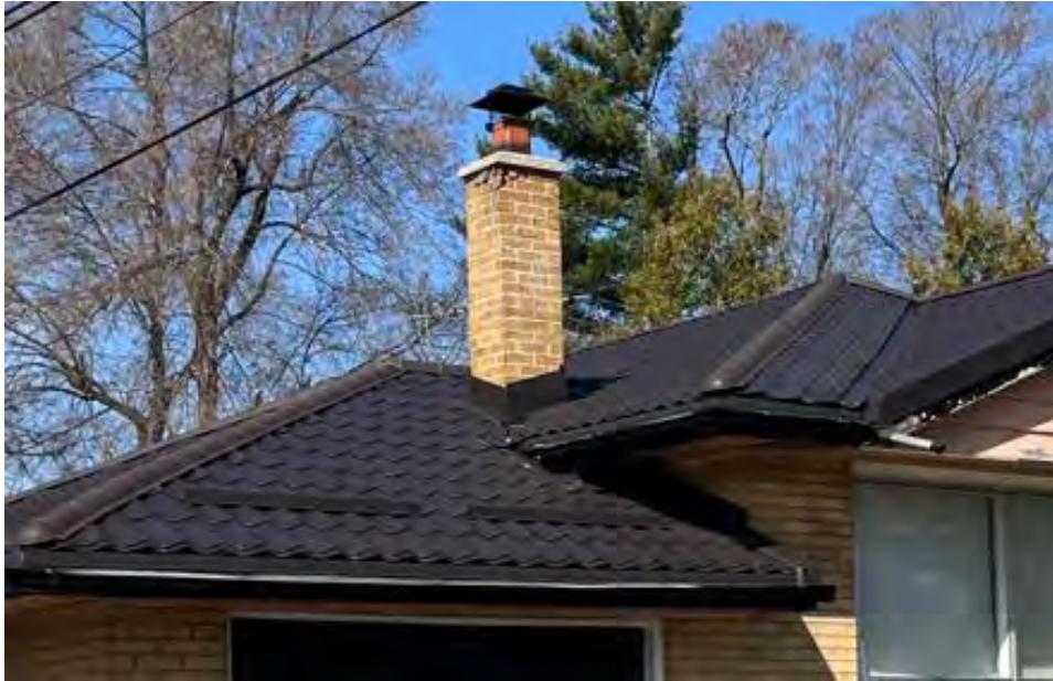
Figure 14: Detail view of the irregular roofline and clay roof-style shingles (A.S.I., 2024).
