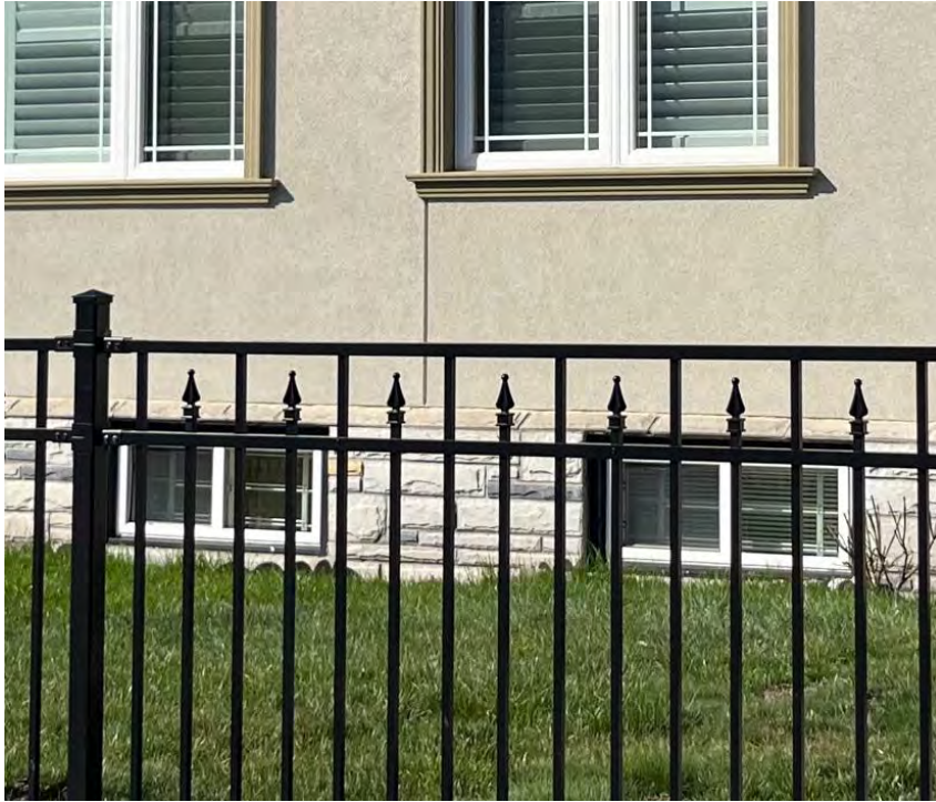
Figure 17: Detail view of angel-stone cladding and basement windows (A.S.I., 2024).
