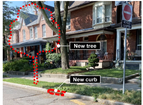
Figure 3: Street view of upgrades on Gladstone Avenue south of Lindsey Avenue
