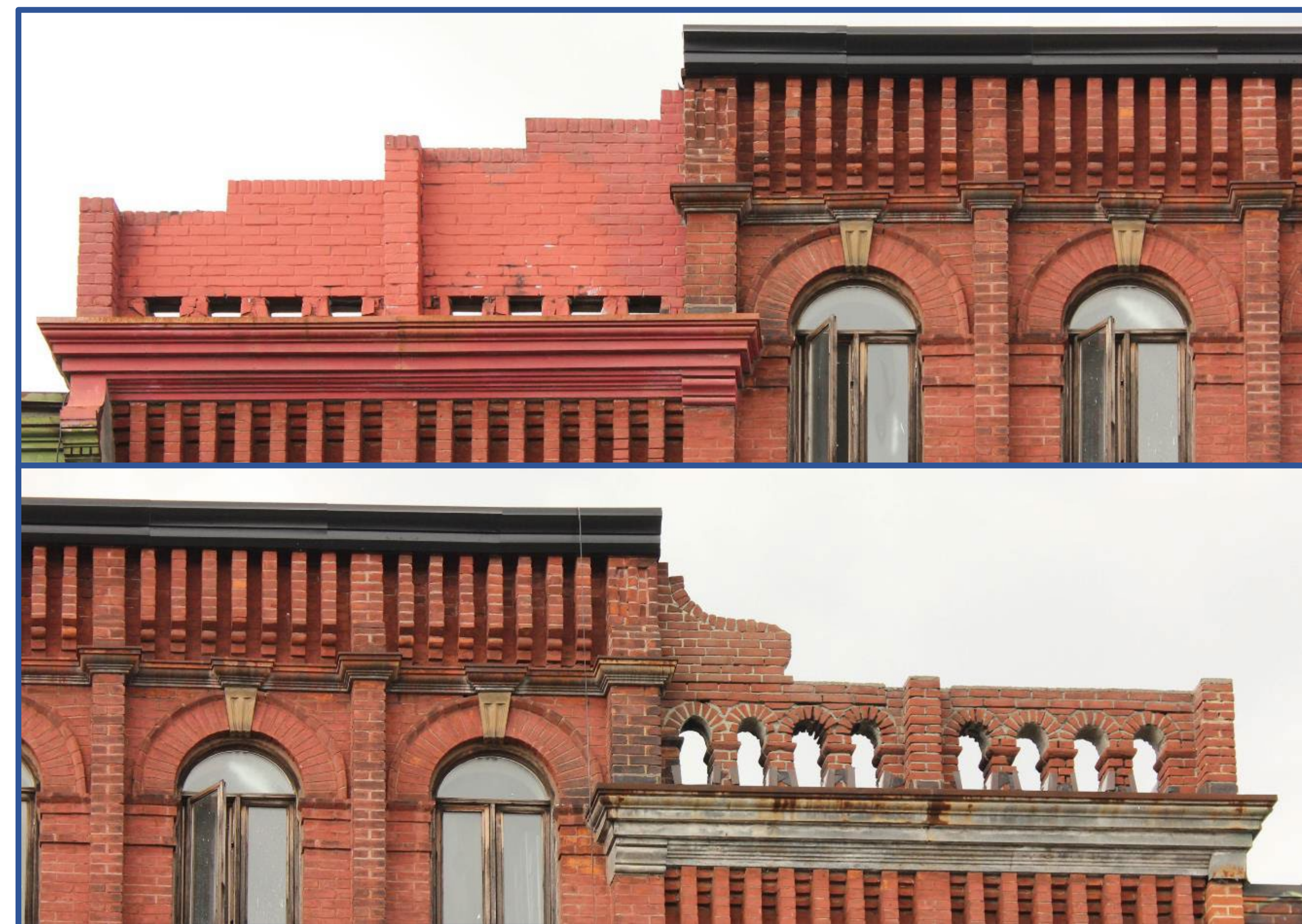
660-664 Queen Street West | Examples of unsympathetic and uneven restoration of the building's parapet
