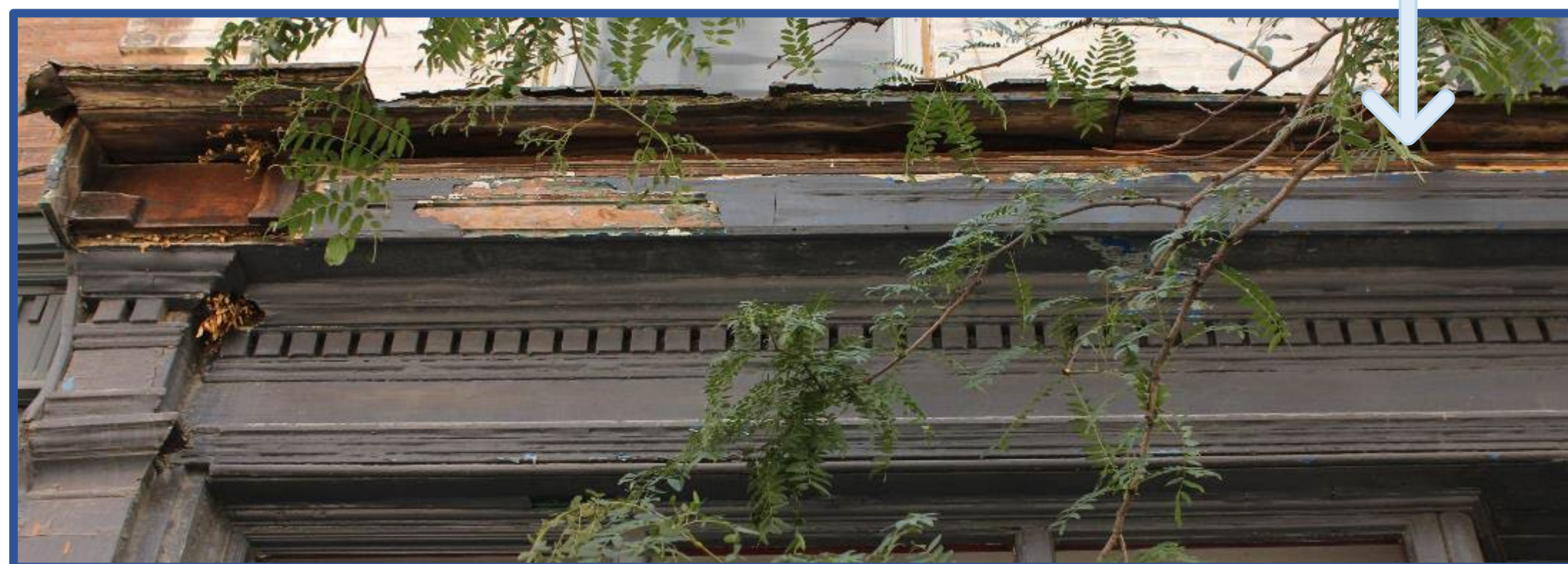
Historic Storefront | Example of wood deterioration in the cornice
