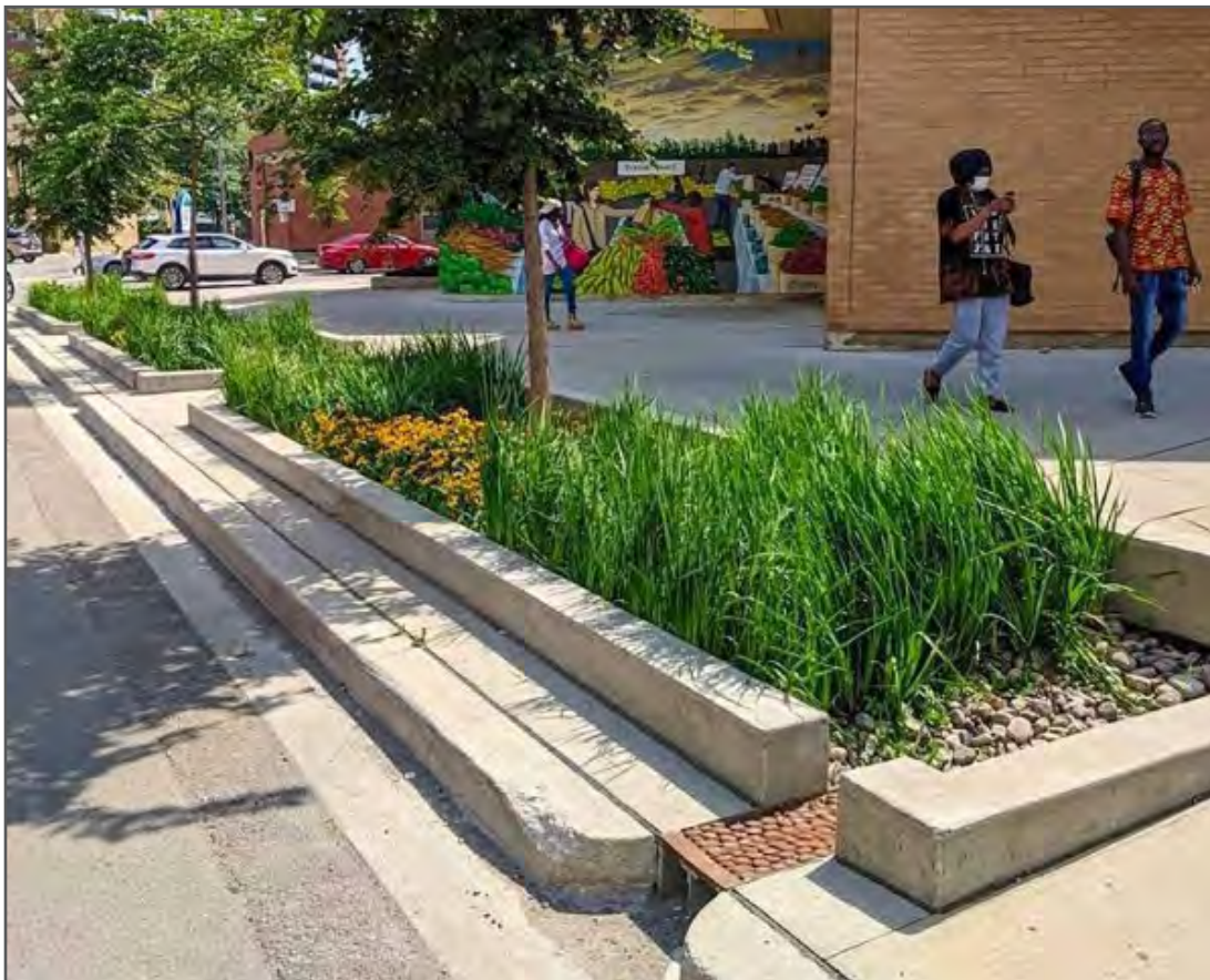
Figure 5-23: Example of a Bioretention Planter, an LID Intervention
