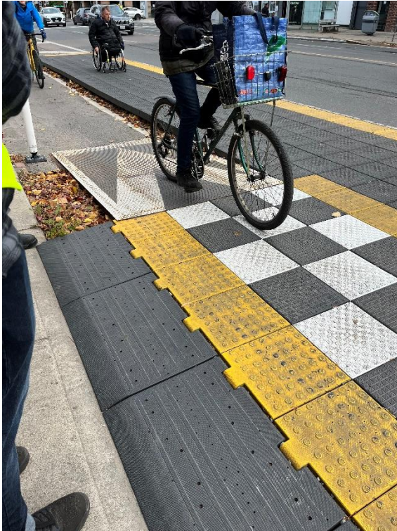
DAVENPORT ROAD AND AVENUE ROAD ZICLA PLATFORM
