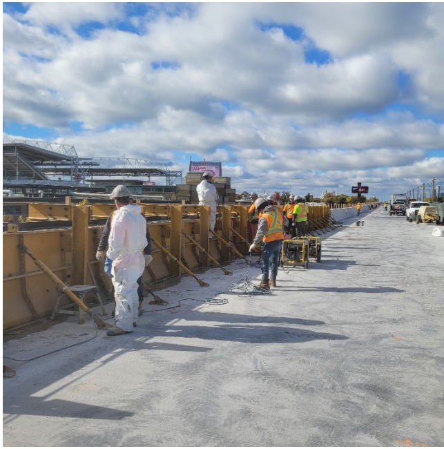
Barrier wall formwork assembly installation
