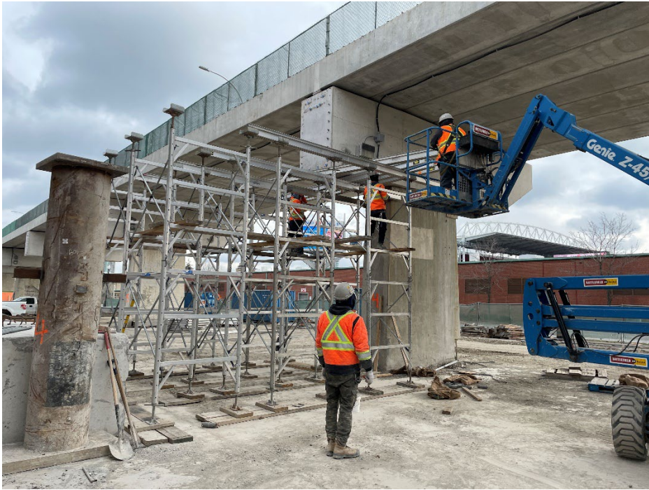
Installation of temporary supports at Bents, west of Exhibition GO.
