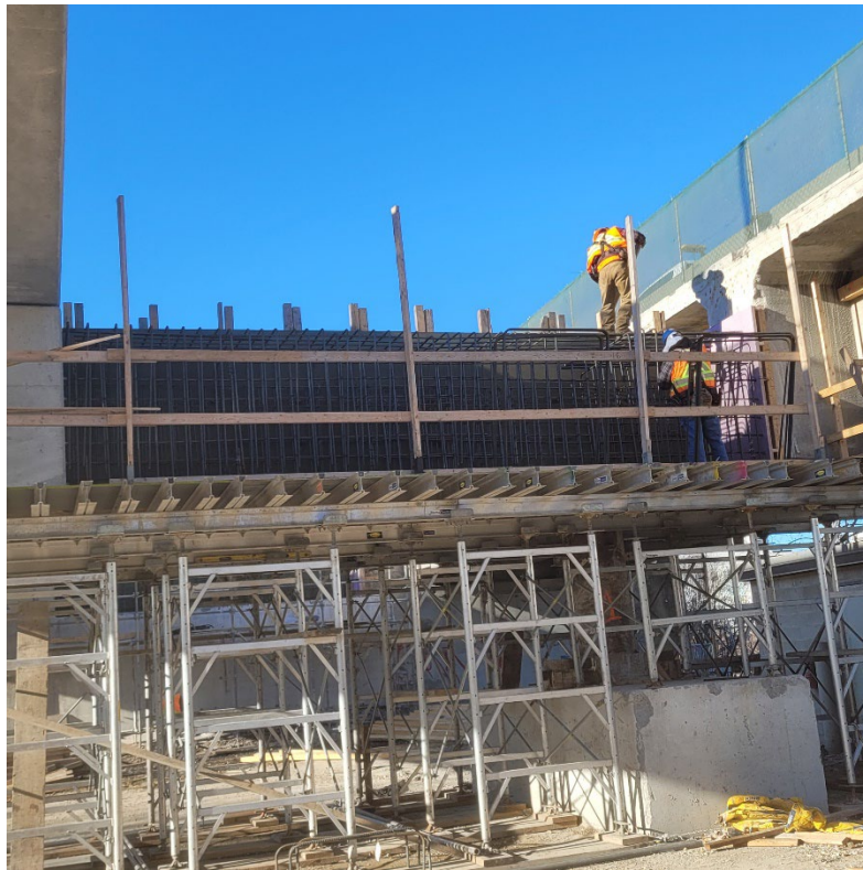
Installation of scaffolding for demolition operation, east of Go Station and TTC loop, Formwork and falsework on Bent 1, 2 and 3.
