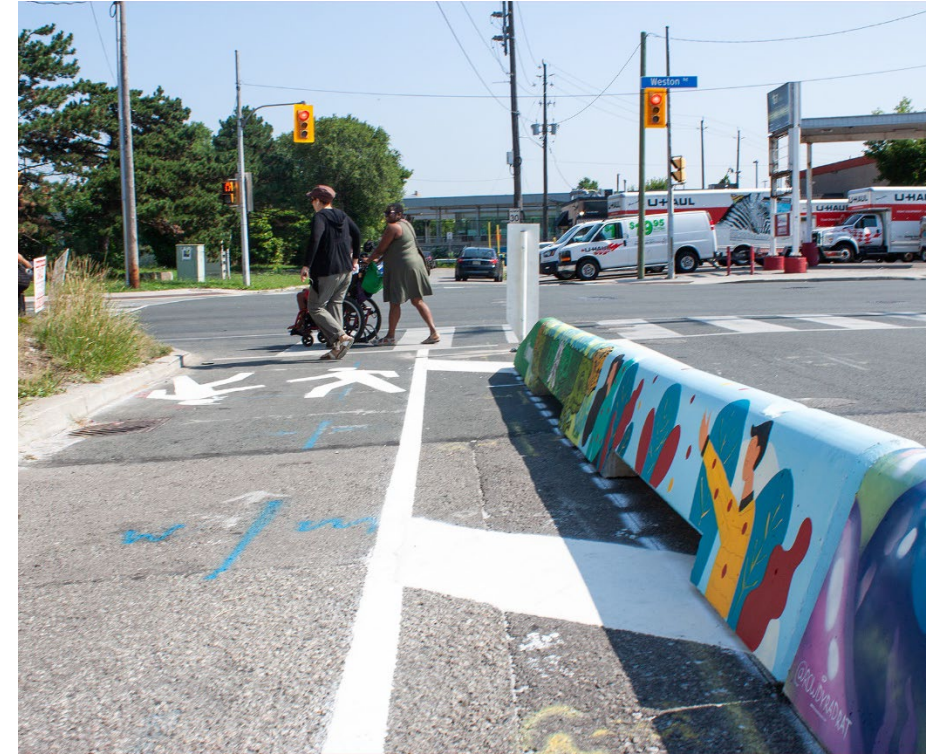
Temporary Sidewalk on Wilby Crescent
