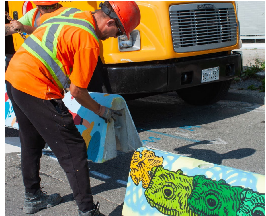
Temporary Sidewalk Installation on Wilby Crescent
