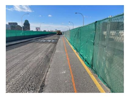
Crews installing green construction screen on top of fence prior to demolition and reconstruction of the roadway.
