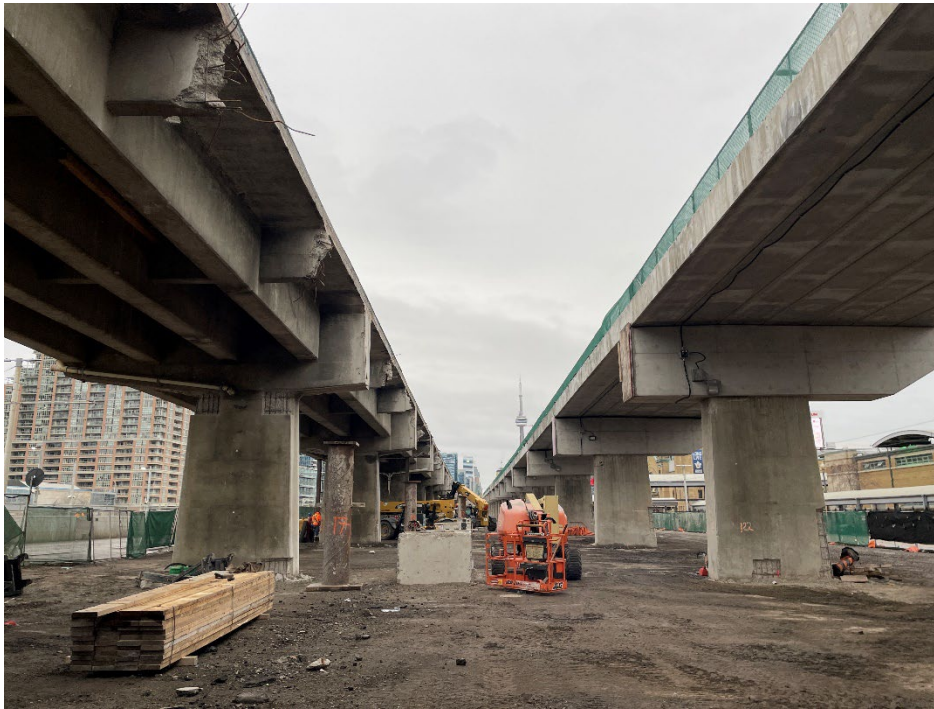
Fully removed steel girders at Stage 2 from Bent 31 to Bent 35.
