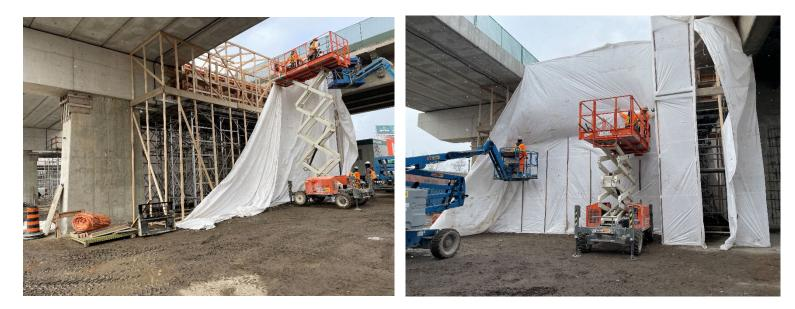
The two images above depict crews setting up the tent enclosure to protect the concrete during cold weather conditions, while the concrete cures. Scaffolding (support system for formwork) for bent cap reconstruction is ongoing.
