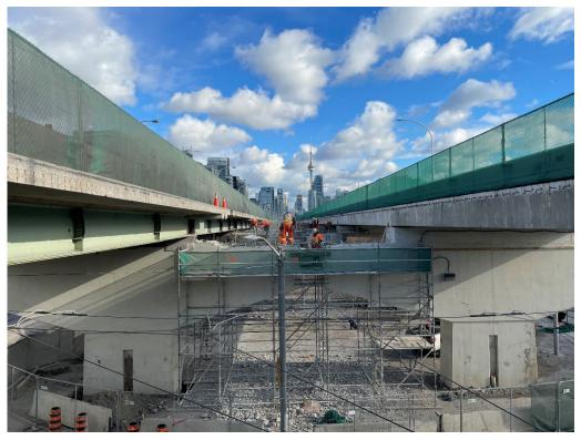
Partial depth removal of Bent caps from Bent 31 to Bent 35 with the use of a hand held chipping tool at the top of the bents.
