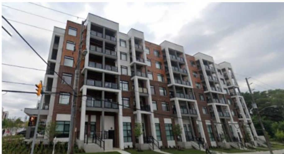
Figure 3.9.3: 120-160 Canon Jackson Drive - Tier 2 TGS Compliant - Key energy performance measures include: High performance building envelope components RSI-7.04/R-40.0 Insulated Roof, RSI-4.40/R-25.0 Fibre Cement Panels.
